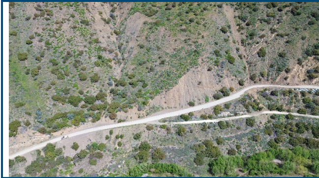
Matilija Canyon Road ~MP 0.5 to 0.7 facing northeasterly
