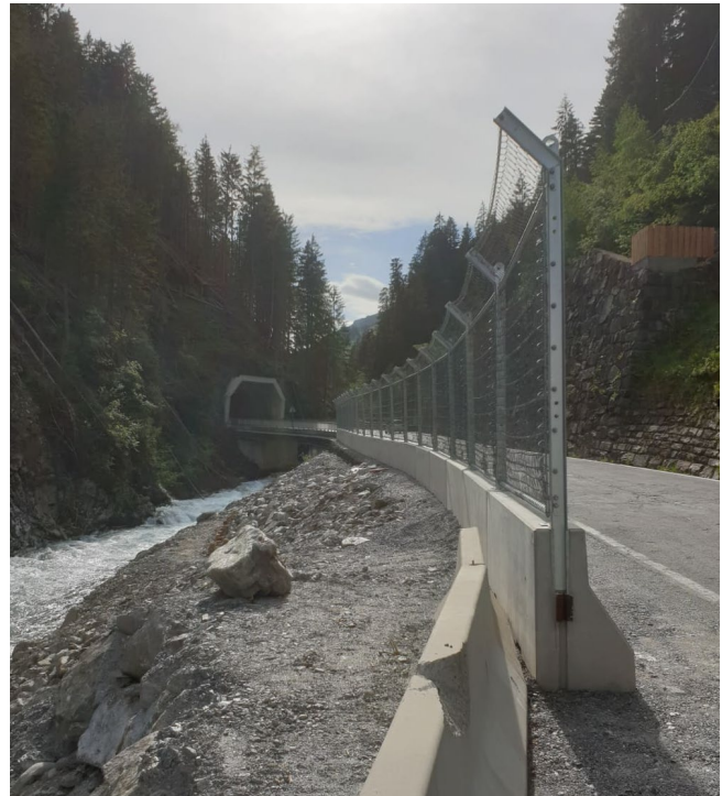
Figure 7: Example of temporary rockfall fence consisting of a debris fence panel embedded into a concrete barrier (credit: Geobrugg)
