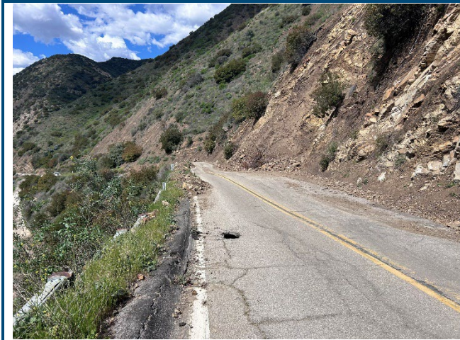
Existing Void, Matilija Canyon Road ~MP 0.53
