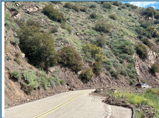
Undermined Matilija Canyon Road and Erosion and Rockfall from above, ~MP 0.58
