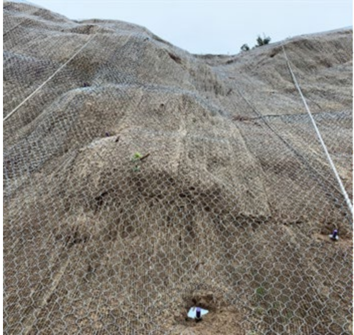
Figure 6: Example of Anchored mesh slope facing prior to hydroseeding
