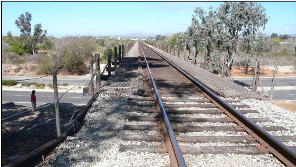
Photo 8. Railroad grade, from south side of Ventura Road, view towards north. [9-18-2014]
