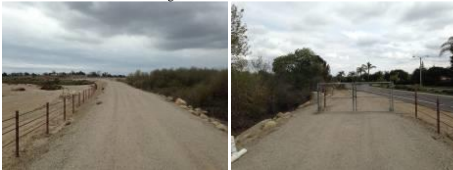
#18-19- Facing NE and SW- at the end of Reach 3
