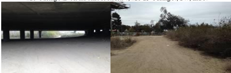
Facing N under the 101 bridge at the end of Reach 4; Facing S- standing near the 101 bridge at the end of Reach 4
