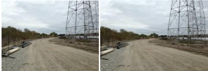
Facing E, toward Victoria Ave. At the start of Reach 1
