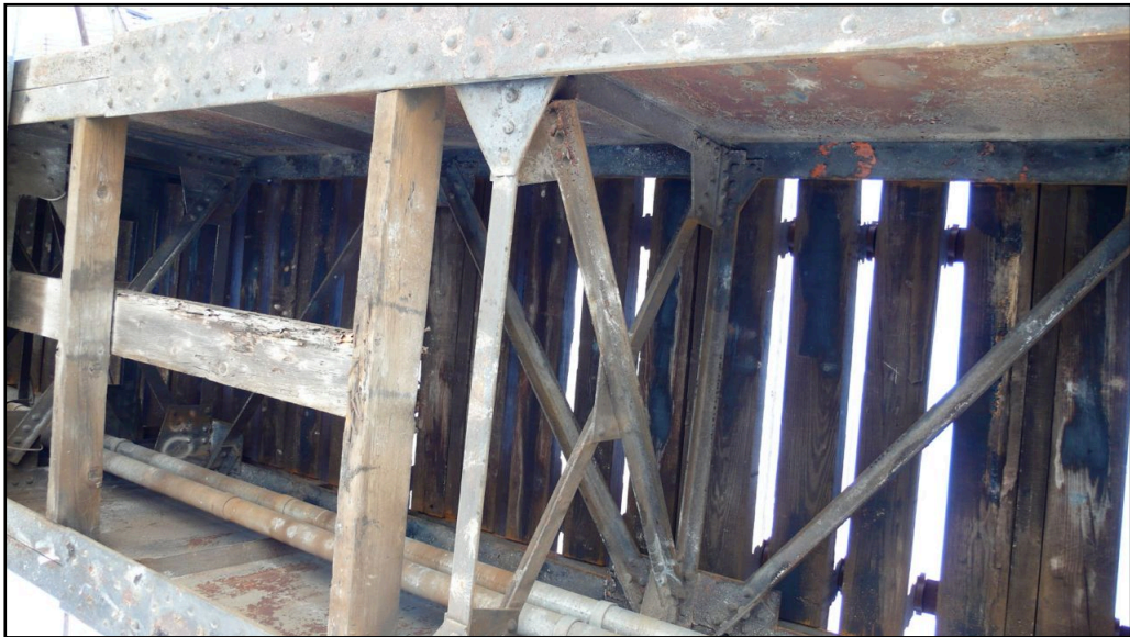
Photo 5. Underside of trestle, typical view of construction methods. [9-18-2014]
