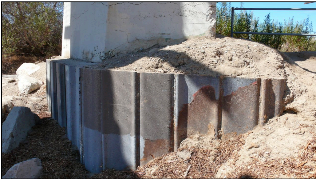
Photo 6. Foot of pier, typical. [9-18-2014]
