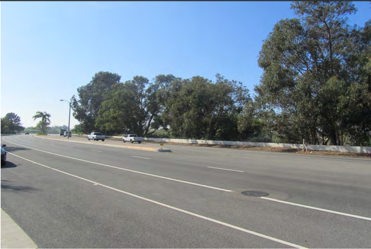
Figure 3.3-2a: Existing view of Reach 4 on N. Ventura Road looking west
