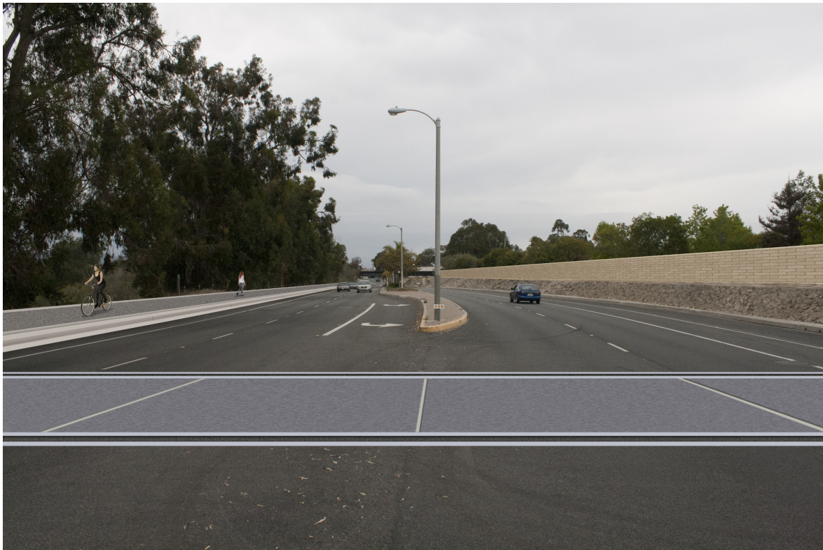
Figure 3.3-1b: Visual simulation looking northeast of the Reach 4 floodwall on the south side (land side) of N. Ventura Road and the flood gate installed within the street (at lowered position)
