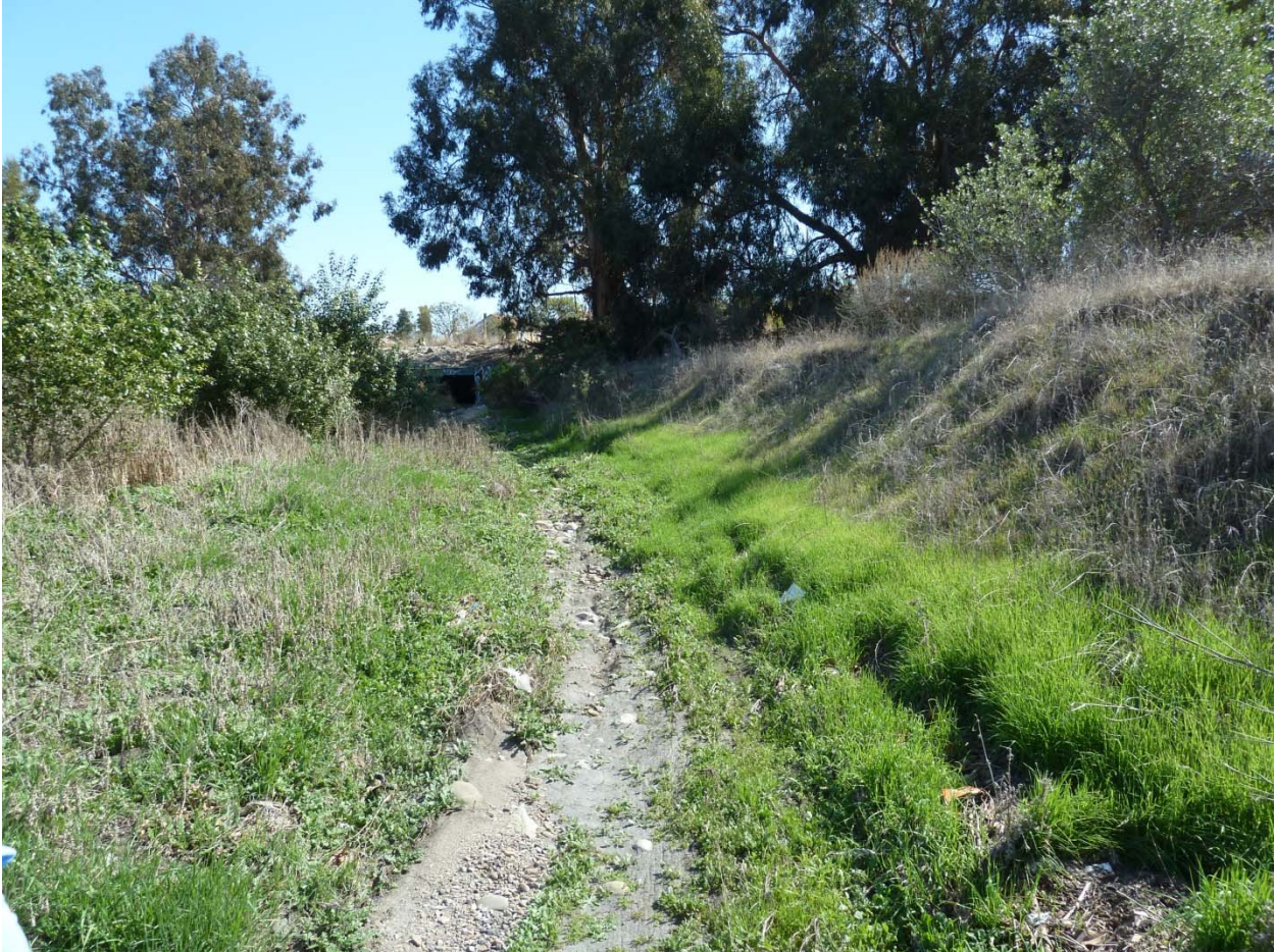
Photo 6 - View looking south, near soil pit El Rio 1, toward the outlet of the culvert under Ventura Road into the El Rio Drainage Channel.
