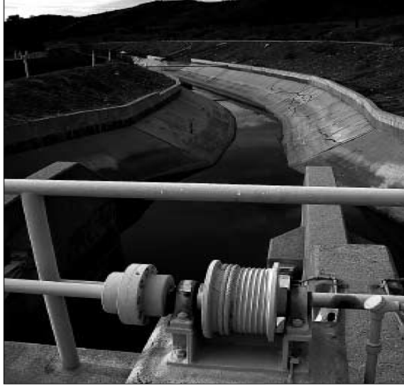
The Robles Diversion Canal carries water from the Ventura River to Lake Casitas.
