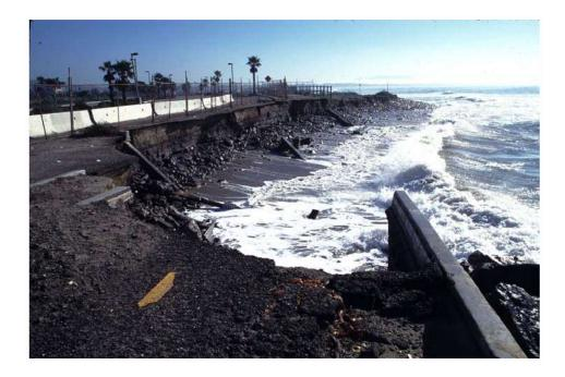
Figure 2-20 – Erosion at Surfer's Point Near Mouth of the Ventura River
