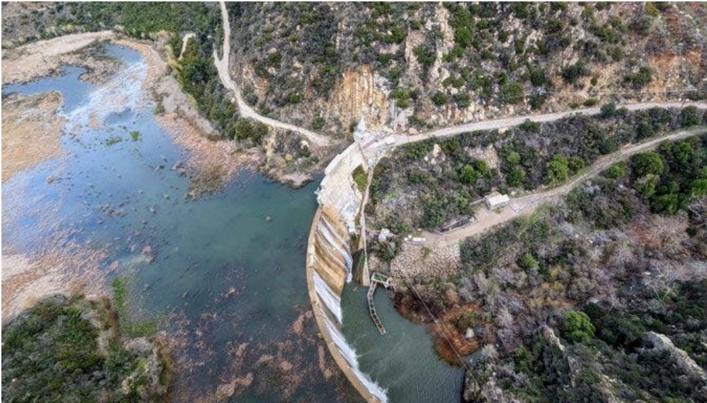
Matilija Dam as seen from a Ventura County Sheriff's helicopter Wednesday morning, Jan. 4, 2023. Two copters from the air unit flew over local watersheds to scout potential issues in advance of an incoming rainstorm. CONTRIBUTED PHOTO/VENTURA COUNTY AIR UNIT
