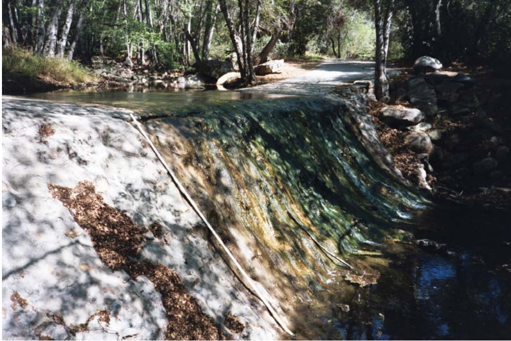
Barrier #710 in Lower North Fork. See Figure 6 for location and Table 2 for barrier details.
