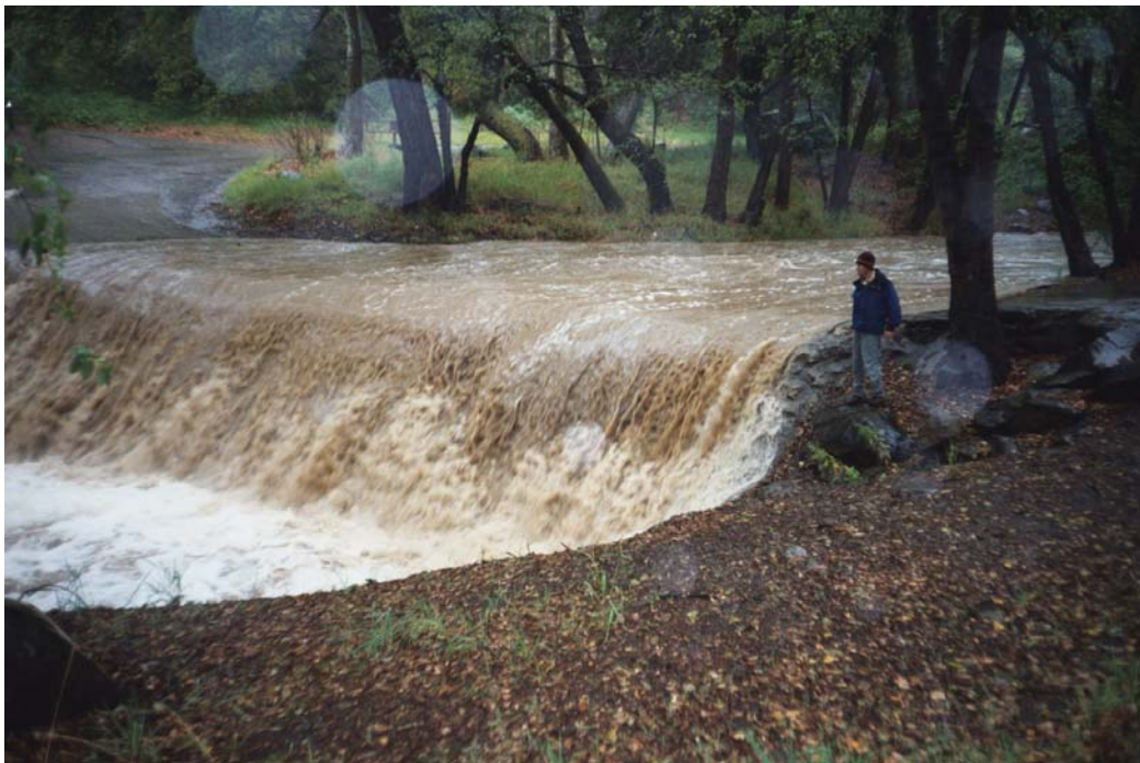
Barrier #710 in Lower North Fork during 15 March storm event. See Figure 6 for location and Table 2 for barrier details.
