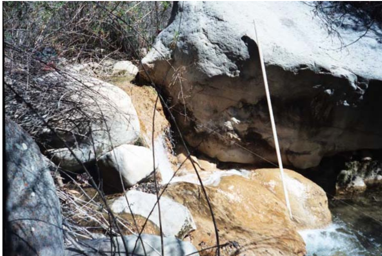
Barrier #74 in Old Man Creek. Visible portion of stadia rod is approximately 9 ft long. See Figure 3 for location and Table 2 for barrier details.
