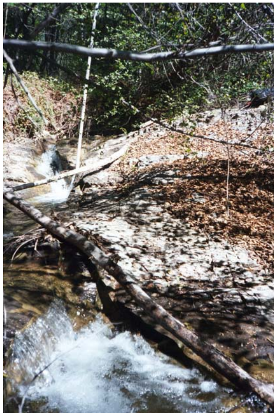
Barrier #49 (left side) in Upper North Fork Matilija Creek. Visible portion of stadia rod is approximately 13 ft long. See Figure 3 for location and Table 2 for barrier details.
