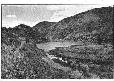
The reservoir behind Matilija Dam is clogged with dirt and sand.
