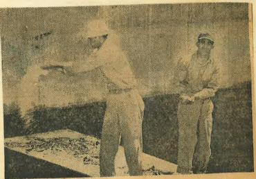
FINISHING TOUCH—Matilija dam workers fling the last bit of salt into reservoir waters as they wind up the first portion of the newest leakage test on the dam. Yesterday, 300 pounds of coarse salt was dissolved in the dam waters by dragging salt-loaded bags back and forth through the water. Now, water samples are being taken at grout holes near J, K and L blocks to determine the salt content and to see if the salt-treated water is leaking through or under the dam.
