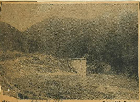
Photo by Midge Mossberg stretching be into the canyon area. This scene shows the dam with about 250 acre feet of water sowed. 300 ainds of coarse salt as a new test was started to determine leakage of the dam's foundation.
