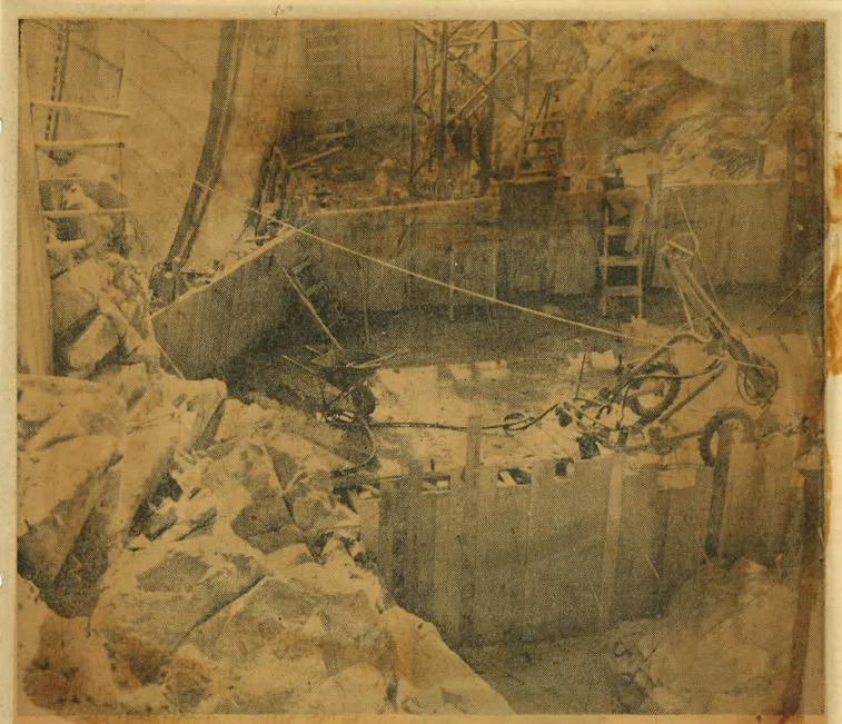
POURING OF THRUST BLOCKS—Shown above is the pouring of thrust blocks on the left abutment after considerable excavation to remove clay seams found beneath rock. The operation delayed considerably the progress of the dam, but contractors were
