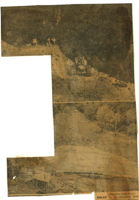
DELAY — A rainstorm that flooded the damsite in Matilija canyon before the first blocks were poured. The forms had been constructed and pouring was nearly ready to begin when the flash flood jumped a coffer dam upstream and came pouring into the excavation, inun-
