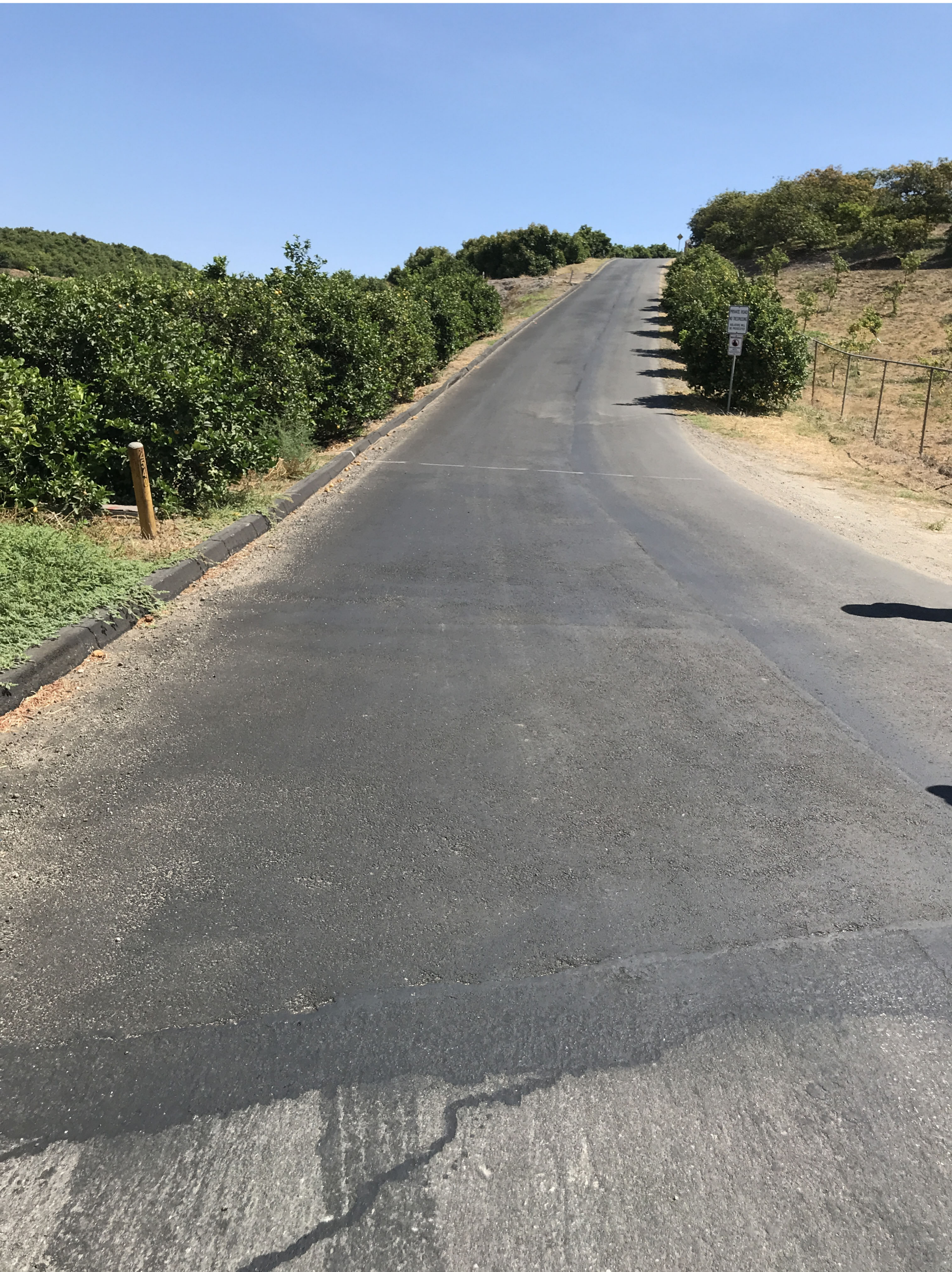
Recently slurry sealed portion of Worth Way.
