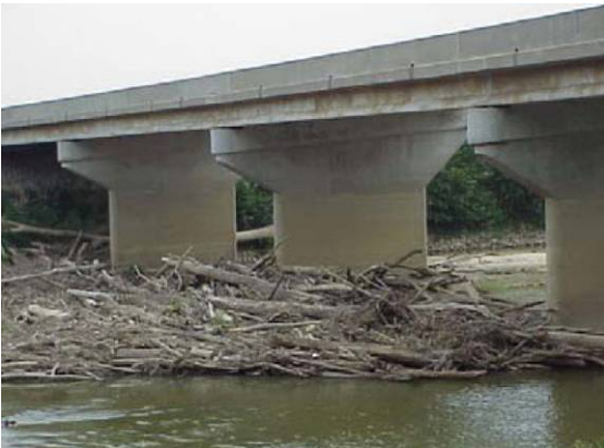
Figure 9-1. Woody Debris Blocking the Waterway Opening of the Bridge (Lyn et al., 2003)
