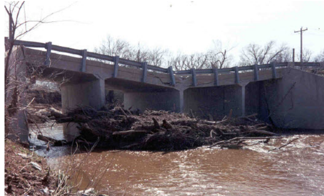
Figure 9-2. Woody Debris Accumulation and Bridge Failure (FHWA, 2005)
