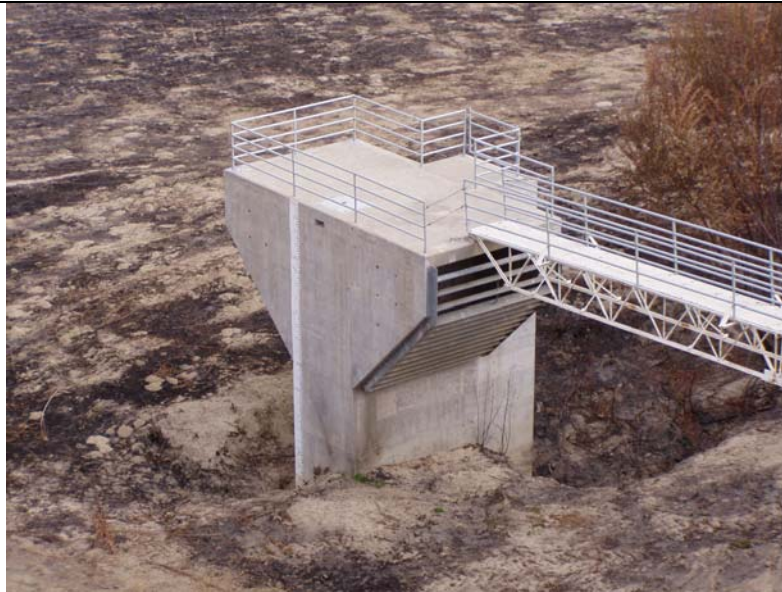
Las Lllajas Detention Basin- Zone 3. Operating Spillway, Reinforced Concrete Riser Tower with Projecting Top and Side Inlets with Trash Rack
