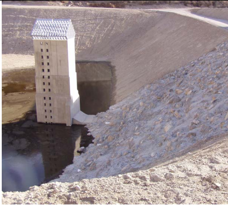
Warring Canyon Debris Basin- Zone 2. Operating Spillway- Riser Tower with Debris Bleeder Orifice Inlets and Weir Inlet Top Protected with Inclined Trash Rack
