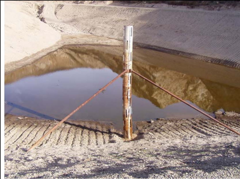
Real Wash Debris Basin- Zone 2. Perforated CMP Debris Bleeder Riser Tower
