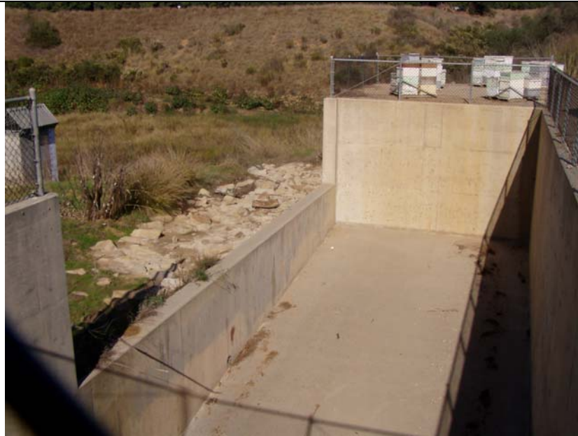
Ferro Debris Basin- Zone 3. Emergency Spillway- Side Inlet Drop Box (riser tower in the background)
