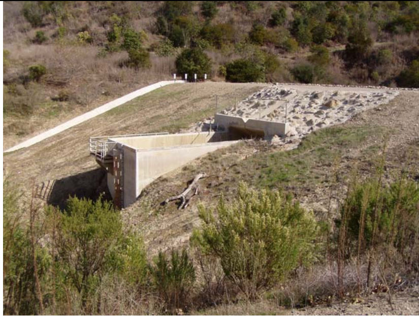
Adams Wash Debris Basin- Zone 2. Emergency Spillway, Three-Sided Drop Box Inlet (with attached perforated CMP debris bleeder)
