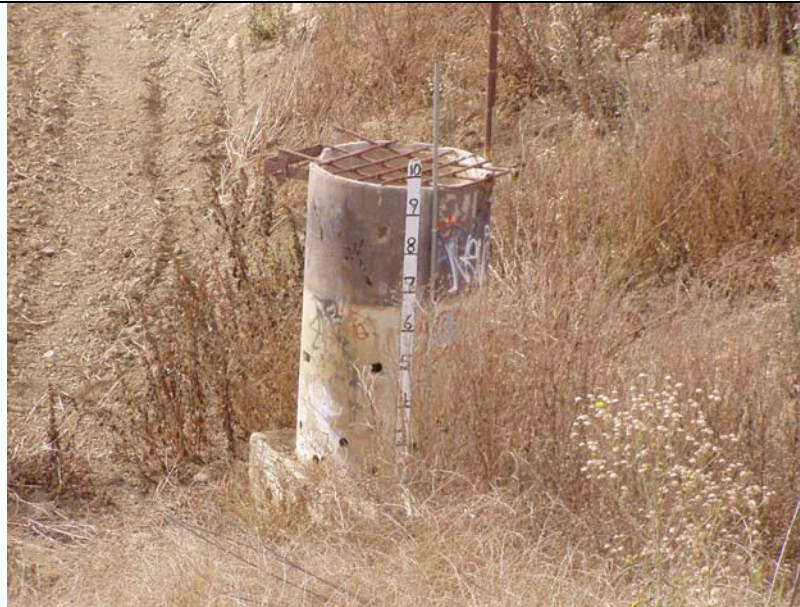
Runkle Detention Basin-Zone 3. Operating Spillway- Perforated 48" RCP Riser with Grated Weir Inlet
