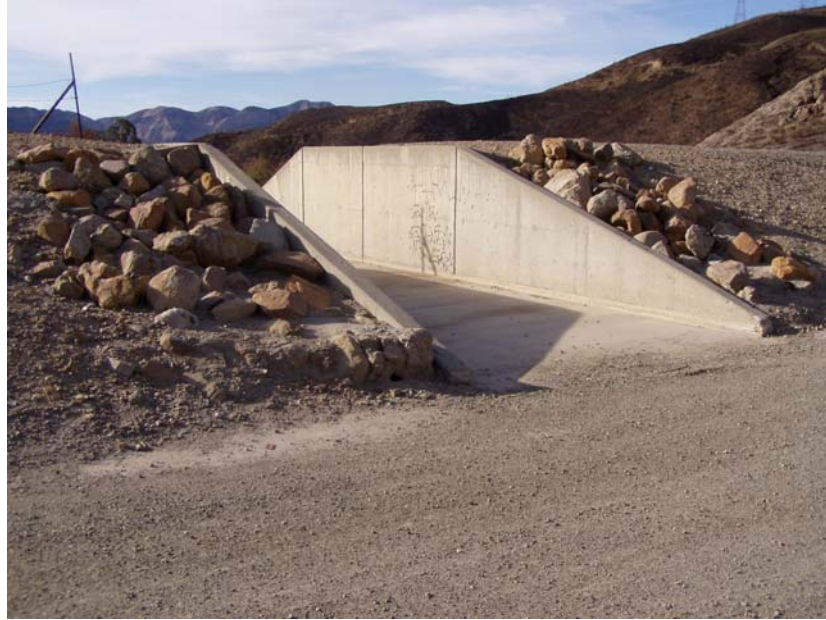
Real Wash Debris Basin- Zone 2. Emergency Spillway: Reinforced Concrete Rectangular Channel
