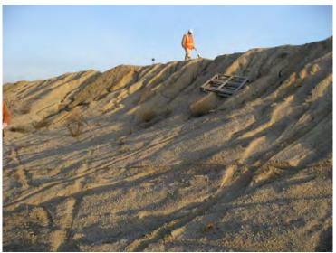
Santa Clara River Levee, From Hwy 101 to Saticoy. (Photo No. M15) – Erosion of levee embankment, looking upstream (riverward side)
