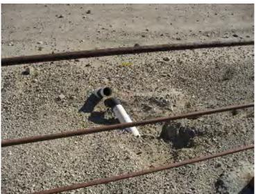
Santa Clara River Levee, From Hwy 101 to Saticoy, (Photo No. M43) – PVC pipe protruding from levee (landward side)
