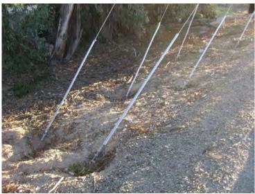
**Santa Clara River Levee,** *From Hwy 101 to Saticoy,* (Photo No. M63) – Power poles guy wires anchored in levee bank, looking d/s (landward side)
