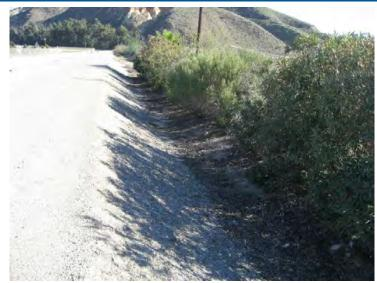
**Santa Clara River Levee,** *From Hwy 101 to Saticoy*, (Photo No. M81) – Vegetation within 15-feet of levee toe, looking upstream (landward side)
