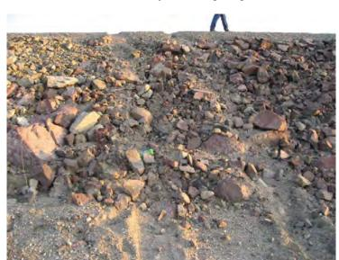
Santa Clara River Levee, From Hwy 101 to Saticoy. (Photo No. M18) – Levee embankment erosion caused by vehicles (riverward side)
