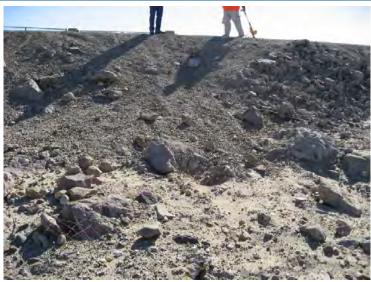
Santa Clara River Levee, From Hwy 101 to Saticoy. (Photo No. M31) – Sloughing levee embankment protection (riverward side)
