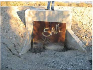
Santa Clara River Levee, From Hwy 101 to Saticoy, (Photo No. M71) – Sediment & metal debris in Side Drain No. 3 inlet (landward side)
