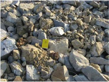
Santa Clara River Levee, From Hwy 101 to Saticoy. (Photo No. M8) – Broken stone revetment (riverward side)
