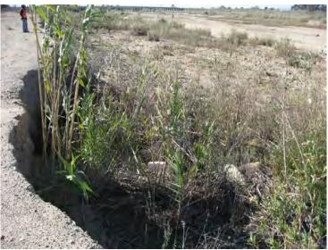
Santa Clara River Levee, From Hwy 101 to Saticoy. (Photo No. M35) – Exposure of tip of buried groin looking downstream (riverward side)
