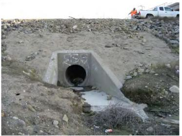
**Santa Clara River Levee,** *From Hwy 101 to Saticoy.* (Photo No. P3) – Side Drain No. 2, 48" RCP located just U/S of L.A. Ave. (riverward side)
