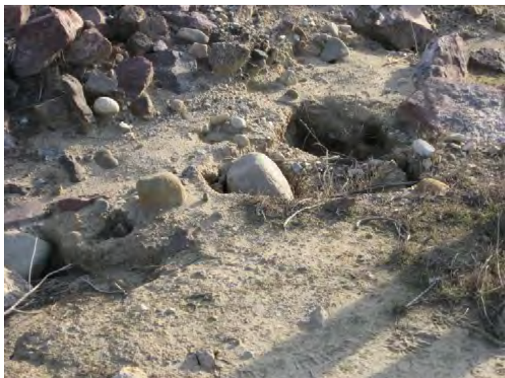
Santa Clara River Levee, From Hwy 101 to Saticoy. (Photo No. M10) – Animal burrows at levee toe (riverward side)
