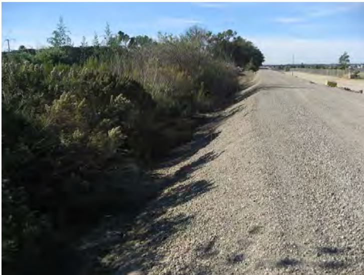
Santa Clara River Levee, From Hwy 101 to Saticoy, (Photo No. M82) – Vegetation within 15-feet of levee toe, looking downstream (landward side)
