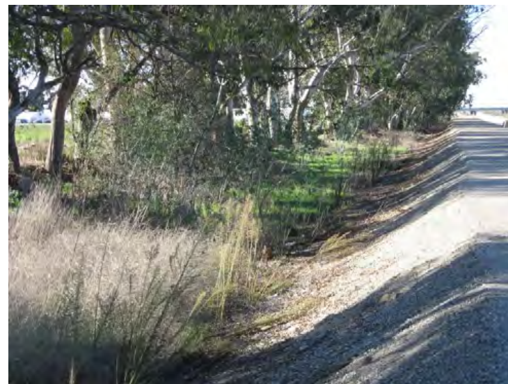
Santa Clara River Levee, From Hwy 101 to Saticoy, (Photo No. M79) – Trees within 15-feet of levee toe, looking downstream (landward side)
