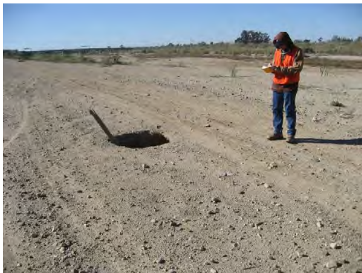
Santa Clara River Levee, From Hwy 101 to Saticoy. (Photo No. M34) – Sink hole in soil covering buried groins looking down/s (riverward side)
