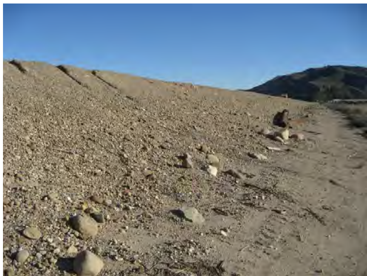
Santa Clara River Levee, From Hwy 101 to Saticoy, (Photo No. M77) – Erosion at top of levee with debris at toe, looking d/s (landward side)
