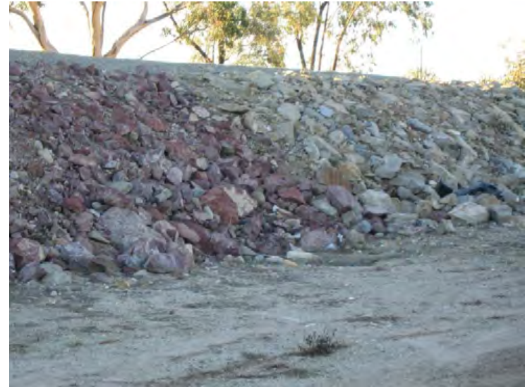
Santa Clara River Levee, From Hwy 101 to Saticoy. (Photo No. F5) – Levee bank stone protection, two different types of stone (riverward side)
