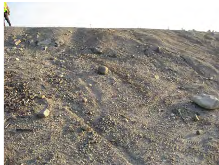
Santa Clara River Levee, From Hwy 101 to Saticoy. (Photo No. M11) – Erosion of levee embankment (riverward side)
