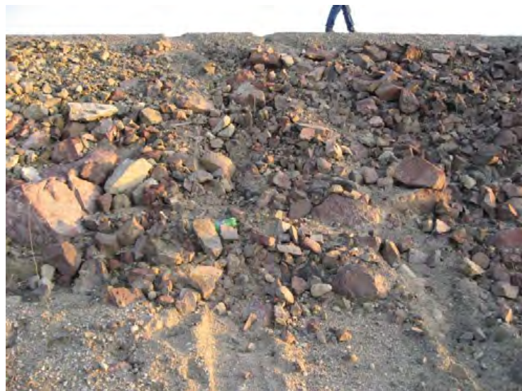
Santa Clara River Levee, From Hwy 101 to Saticoy. (Photo No. M18) – Levee embankment erosion caused by vehicles (riverward side)
