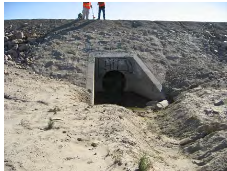
Santa Clara River Levee, From Hwy 101 to Saticoy. (Photo No. P8) – Side Drain No. 6, 48” RCP
