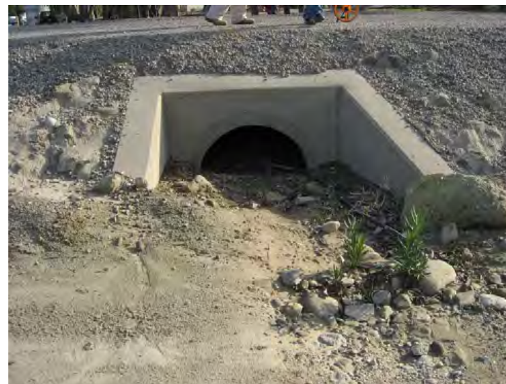
Santa Clara River Levee, From Hwy 101 to Saticoy. (Photo No. M4) – Sediment deposition in Side Drain No. 1, 42" RCP outlet (riverward side)
