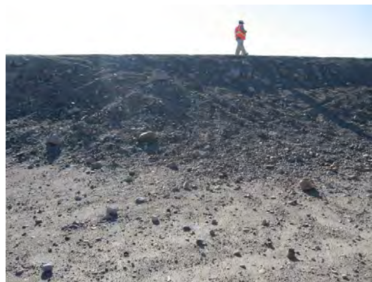
Santa Clara River Levee, From Hwy 101 to Saticoy. (Photo No. M27) – Unauthorized ramp on levee (riverward side)
