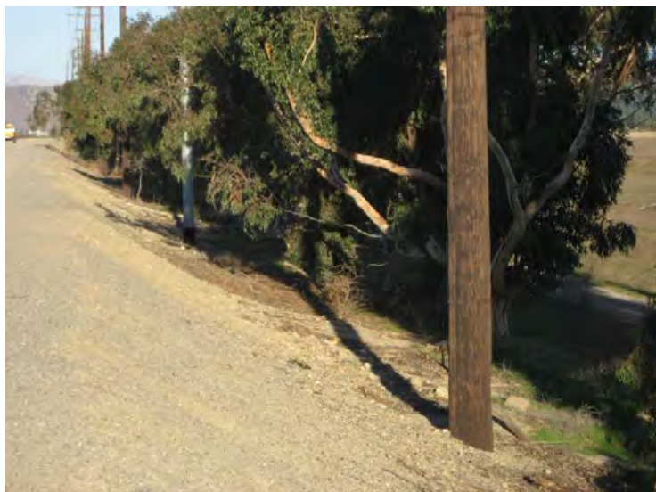
Santa Clara River Levee, From Hwy 101 to Saticoy, (Photo No. M58) – Power poles within 15' of levee toe, looking upstream (landward side)
