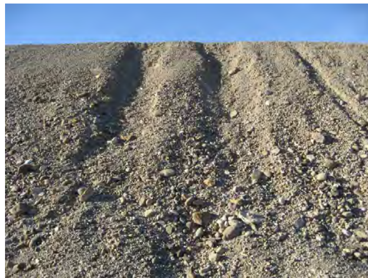
Santa Clara River Levee, From Hwy 101 to Saticoy, (Photo No. M52) – Erosion on levee embankment, looking downstream (landward side)
