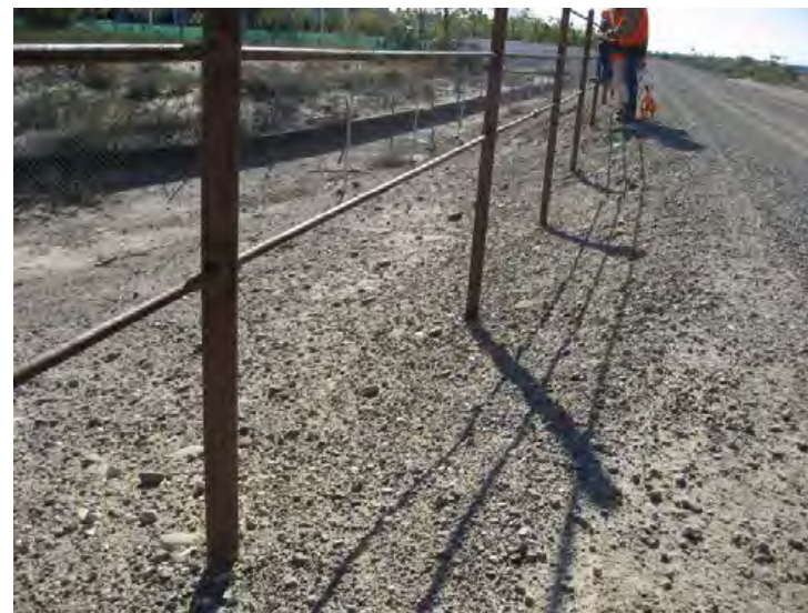
Santa Clara River Levee, From Hwy 101 to Saticoy, (Photo No. M44) – Erosion on top of levee exposing fence posts, looking d/s (landward side)
