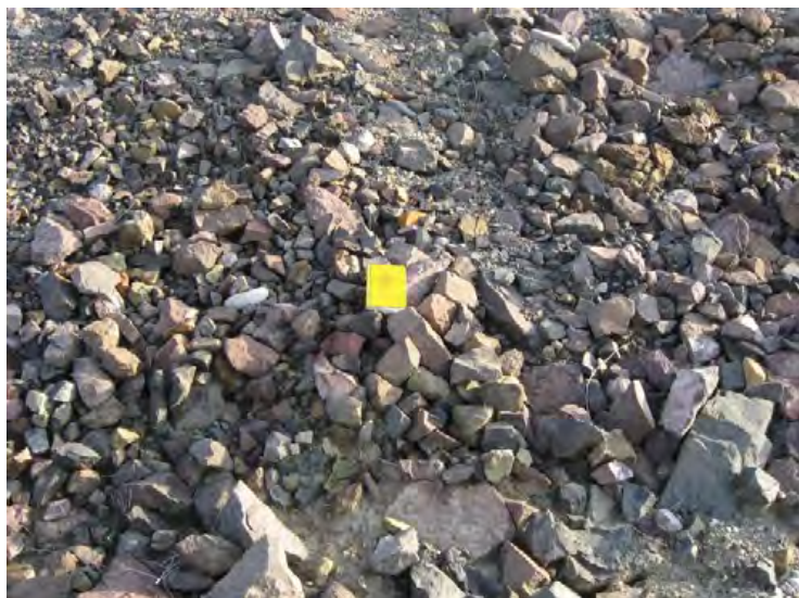
Santa Clara River Levee, From Hwy 101 to Saticoy. (Photo No. M9) – Broken stone revetment (riverward side)
