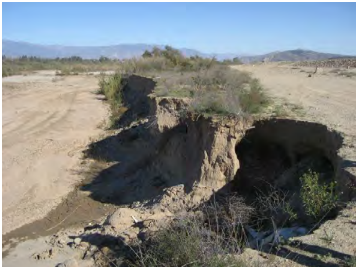
Santa Clara River Levee, From Hwy 101 to Saticoy. (Photo No. F4) – Erosion cut eroding towards levee exposing groins, looking u/s (riverward)
