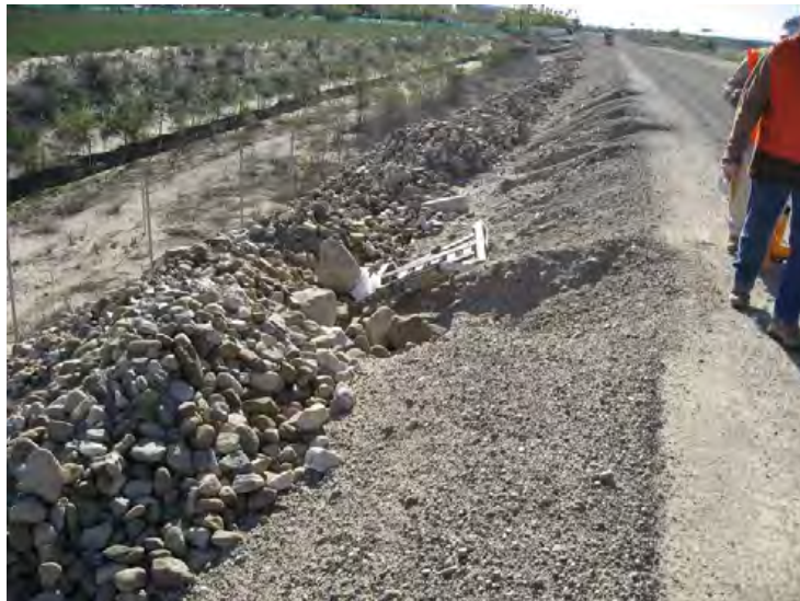
Santa Clara River Levee, From Hwy 101 to Saticoy, (Photo No. M46) – Erosion on top of levee, looking downstream (riverward side)
