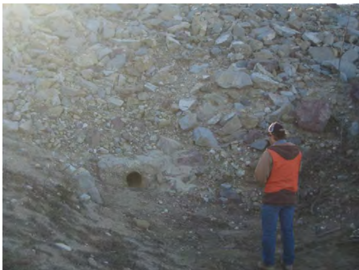
Santa Clara River Levee, From Hwy 101 to Saticoy. (Photo No. P5) – 12” metal pipe, commercial drain from process plant (riverward side)
