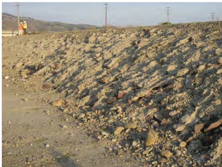
Santa Clara River Levee, From Hwy 101 to Saticoy. (Photo No. M13) – Concrete spread over levee embankment, looking d/s (riverward side)
