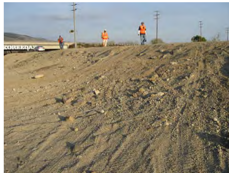
Santa Clara River Levee, From Hwy 101 to Saticoy. (Photo No. M12) – Erosion of levee embankment just downstream of L.A. Ave.(riverward side)
