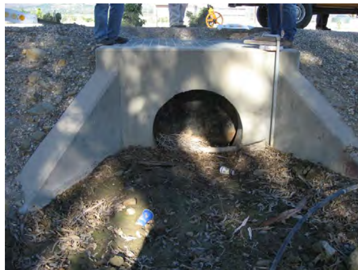
Santa Clara River Levee, From Hwy 101 to Saticoy, (Photo No. M80) – Sediment and debris in Side Drain No.1, 42" RCP inlet (landward side)
