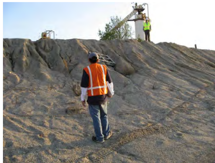
Santa Clara River Levee, From Hwy 101 to Saticoy. (Photo No. M16) – Erosion of levee embankment, adjacent to asphalt plant (riverward side)
