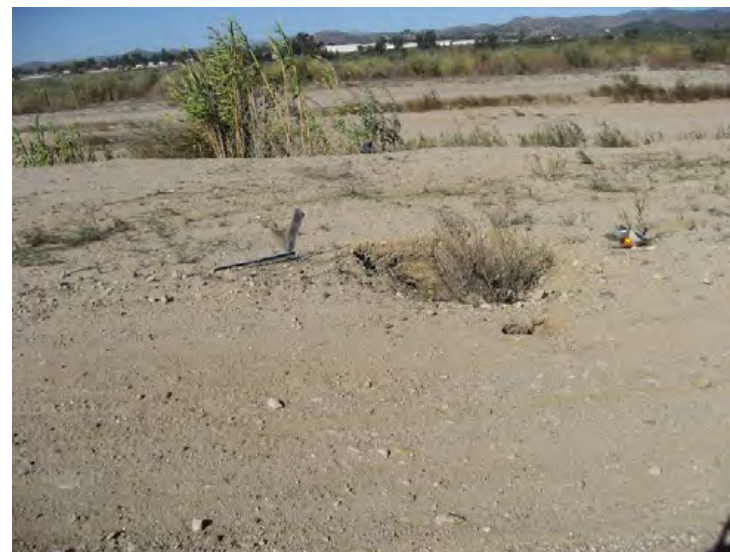
Santa Clara River Levee, From Hwy 101 to Saticoy. (Photo No. M36) – Sink hole in soil covering buried groins (riverward side)
