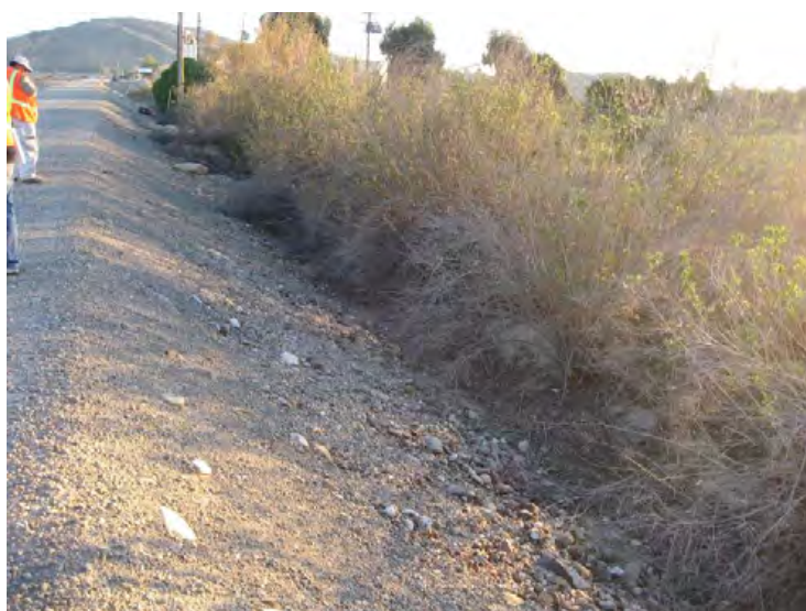
Santa Clara River Levee, From Hwy 101 to Saticoy, (Photo No. M69) – Vegetation within 15-feet of levee toe, looking u/s (landward side)
