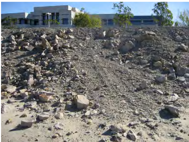
Santa Clara River Levee, From Hwy 101 to Saticoy. (Photo No. M38) – Unauthorized ramp with missing levee embankment protection (riverward)
