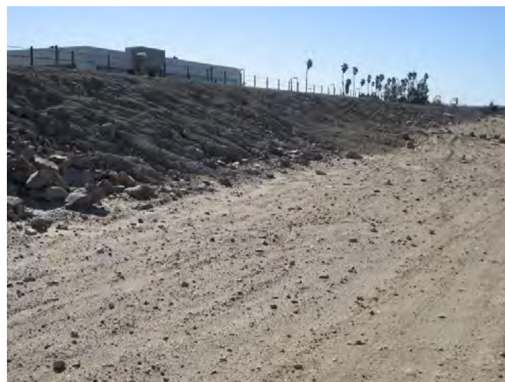
Santa Clara River Levee, From Hwy 101 to Saticoy. (Photo No. M39) – Concrete washout poured over rock protection, looking d/s (riverward side)
