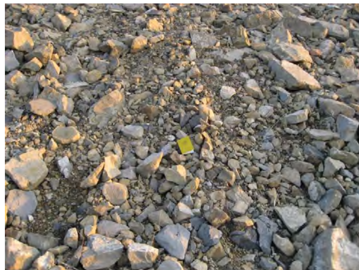
Santa Clara River Levee, From Hwy 101 to Saticoy. (Photo No. M19) – Broken stone revetment (riverward side)
