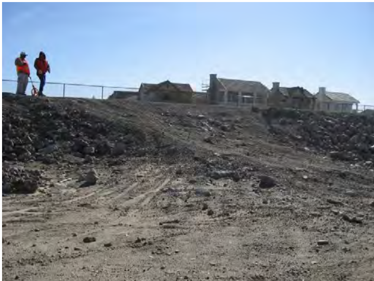
Santa Clara River Levee, From Hwy 101 to Saticoy. (Photo No. M30) – Unauthorized ramp on levee (riverward side)
