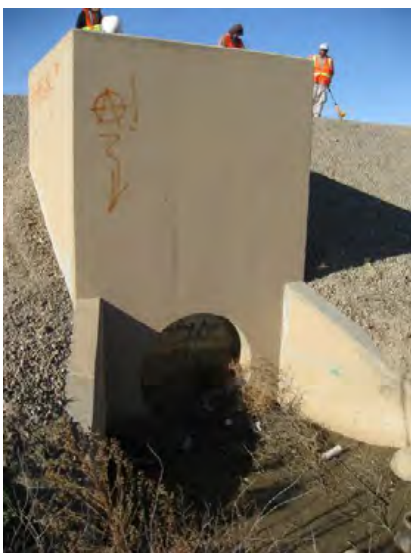
Santa Clara River Levee, From Hwy 101 to Saticoy, (Photo No. M49) – Sediment deposition in Side Drain No. 4, 48" RCP invert (landward side)
