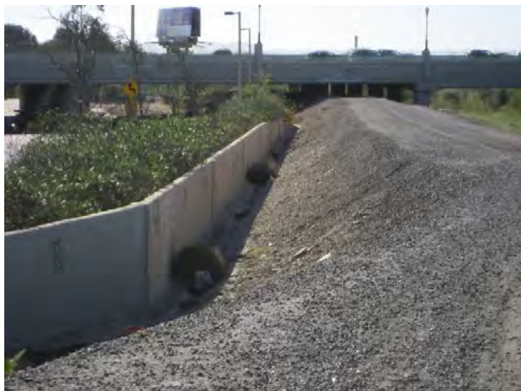
Santa Clara River Levee, From Hwy 101 to Saticoy. (Photo No. M42) – Vegetation within 15-feet of levee toe looking d/s (landward side)
