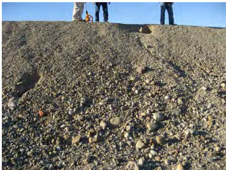
Santa Clara River Levee, From Hwy 101 to Saticoy, (Photo No. M53) – Animal burrows at top of levee (landward side)
