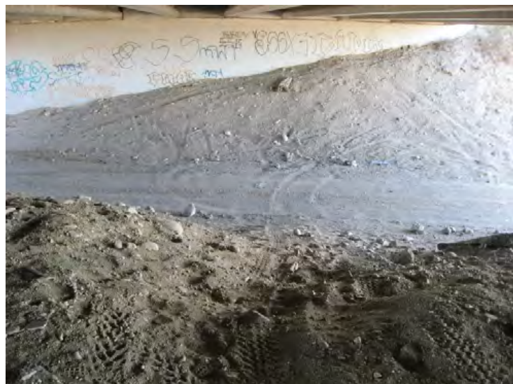
Santa Clara River Levee, From Hwy 101 to Saticoy, (Photo No. M74) – Erosion caused by vehicles under L.A. Ave. Bridge (landward side)
