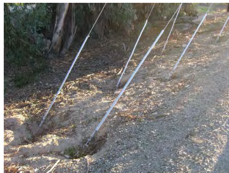
Santa Clara River Levee, From Hwy 101 to Saticoy, (Photo No. M63) – Power poles guy wires anchored in levee bank, looking d/s (landward side)
