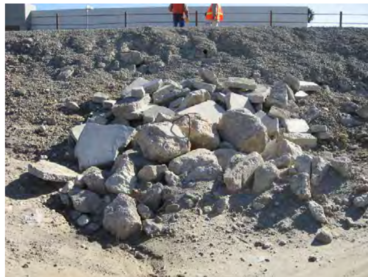
Santa Clara River Levee, From Hwy 101 to Saticoy. (Photo No. M40) – Dumped concrete debris at levee toe (riverward side)
