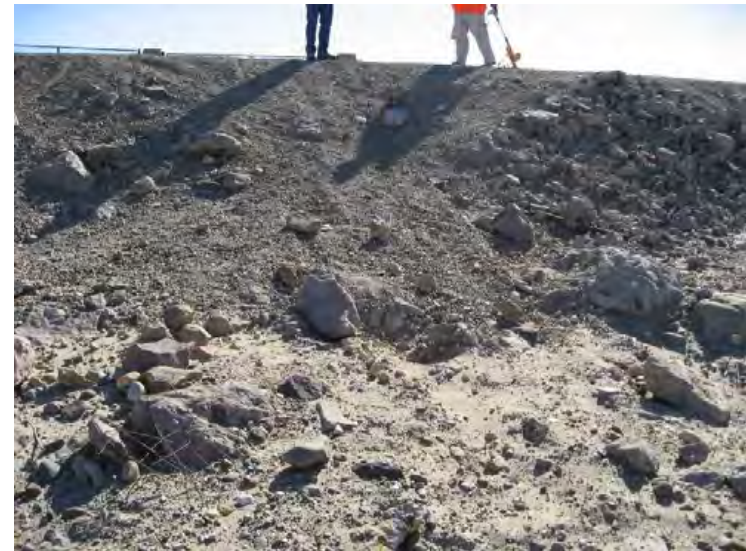
Santa Clara River Levee, From Hwy 101 to Saticoy. (Photo No. M31) – Sloughing levee embankment protection (riverward side)
