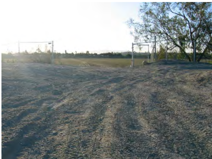
Santa Clara River Levee, From Hwy 101 to Saticoy. (Photo No. M22) – Erosion on top of levee caused by vehicles (riverward side)
