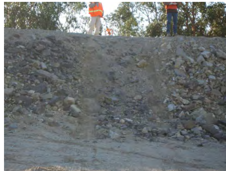
Santa Clara River Levee, From Hwy 101 to Saticoy. (Photo No. M24) – Levee embankment erosion caused by vehicles (riverward side)
