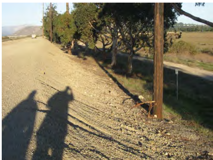
Santa Clara River Levee, From Hwy 101 to Saticoy, (Photo No. M61) – Power poles on levee embankment, looking upstream (landward side)
