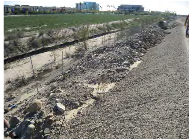
Santa Clara River Levee, From Hwy 101 to Saticoy, (Photo No. M48) – Debris approx. 100' along levee, looking u/s (riverward side)
