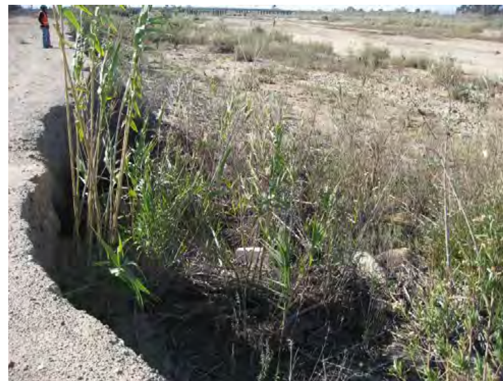
Santa Clara River Levee, From Hwy 101 to Saticoy. (Photo No. M35) – Exposure of tip of buried groin looking downstream (riverward side)
