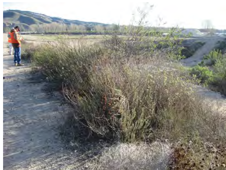
Santa Clara River Levee, From Hwy 101 to Saticoy, (Photo No. M75) – Vegetation within 15-feet of levee toe, looking downstream (landward side)
