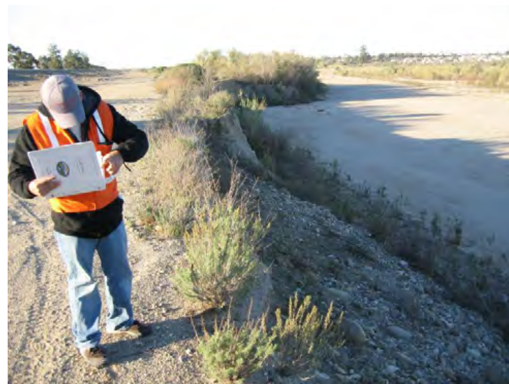
Santa Clara River Levee, From Hwy 101 to Saticoy. (Photo No. F1) – 20' -25' high erosion cut eroding towards levee, looking d/s (riverward)
