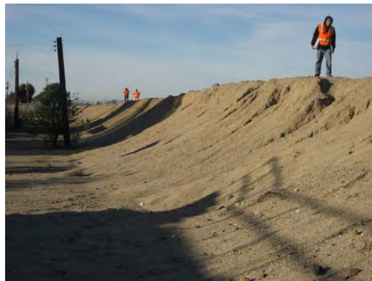
Santa Clara River Levee, From Hwy 101 to Saticoy, (Photo No. M72) – Erosion on levee embankment, looking downstream (landward side)
