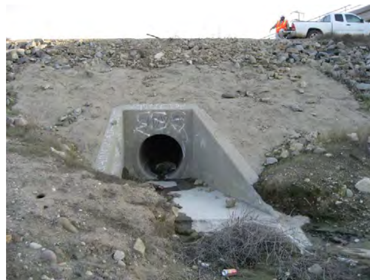
Santa Clara River Levee, From Hwy 101 to Saticoy. (Photo No. P3) – Side Drain No. 2, 48\"/>
