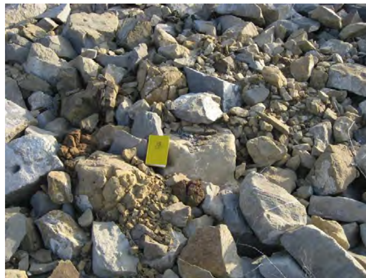
Santa Clara River Levee, From Hwy 101 to Saticoy. (Photo No. M8) – Broken stone revetment (riverward side)
