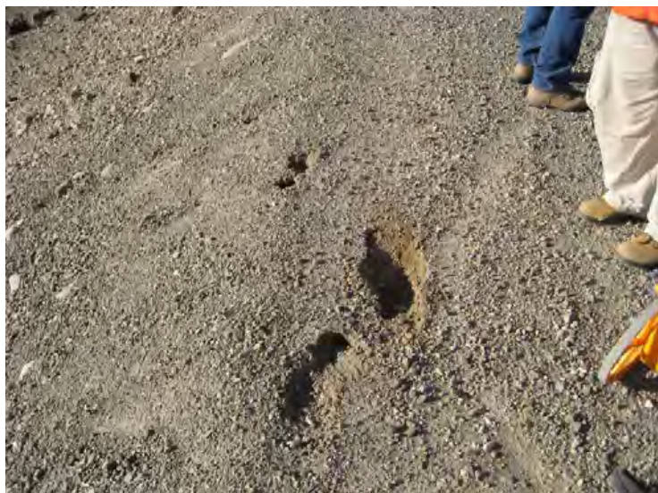
Santa Clara River Levee, From Hwy 101 to Saticoy, (Photo No. M78) – Animal burrows at top of levee (landward side)
