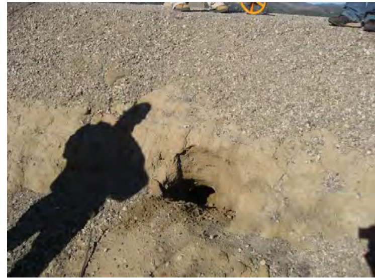
Santa Clara River Levee, From Hwy 101 to Saticoy, (Photo No. M83) – Animal burrows at levee toe (landward side)
