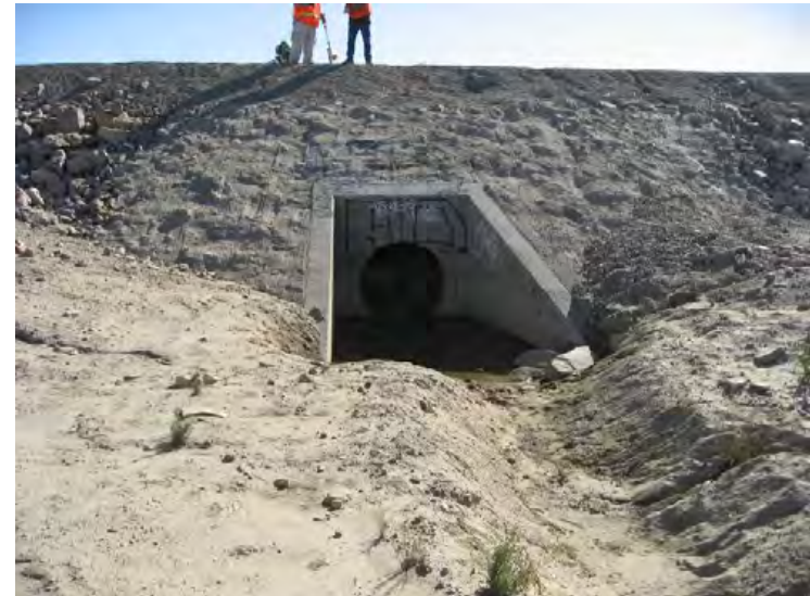
Santa Clara River Levee, From Hwy 101 to Saticoy. (Photo No. M32) – Sediment deposition in Side Drain No. 4, 48" RCP outlet (riverward side)
