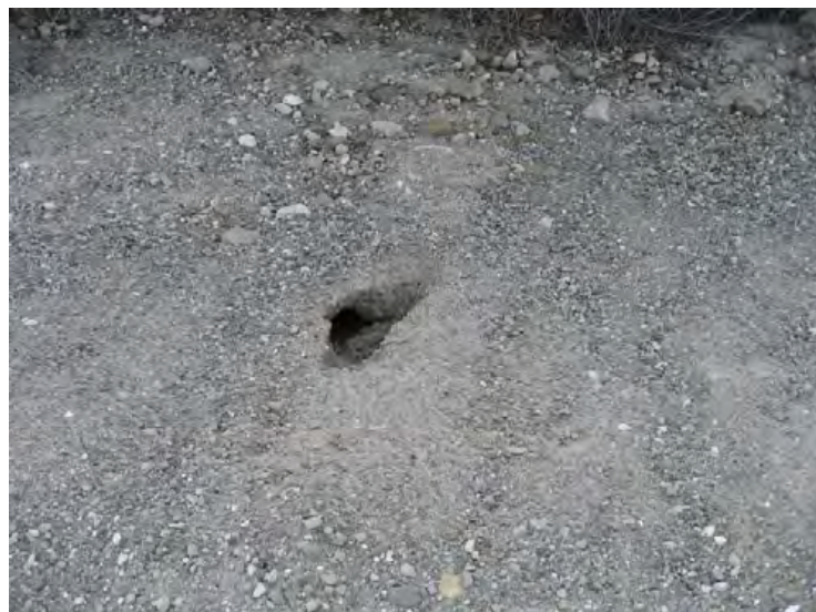
Santa Clara River Levee, From Hwy 101 to Saticoy, (Photo No. M70) – Animal burrow on top of levee (landward side)
