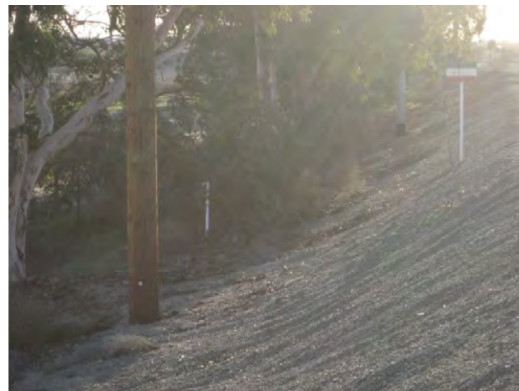
Santa Clara River Levee, From Hwy 101 to Saticoy, (Photo No. M55) – Trees within 15' of levee toe, looking downstream (landward side)
