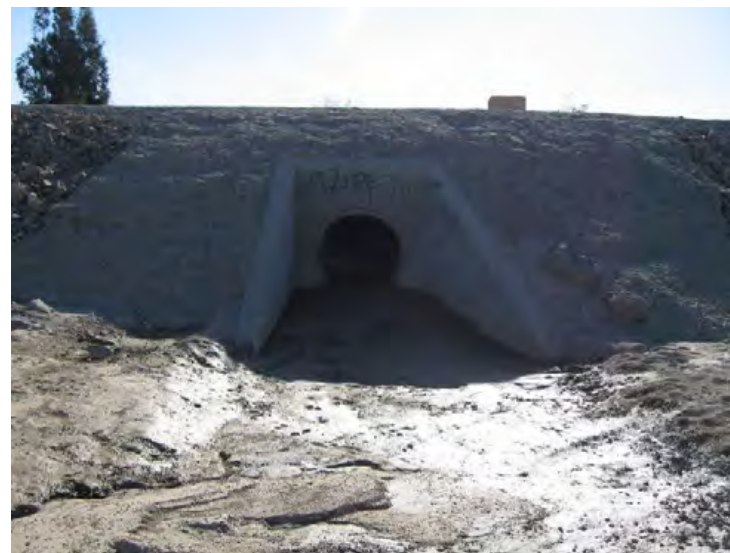
Santa Clara River Levee, From Hwy 101 to Saticoy. (Photo No. P7) – Side Drain No. 4, 48” RCP (riverward side)
