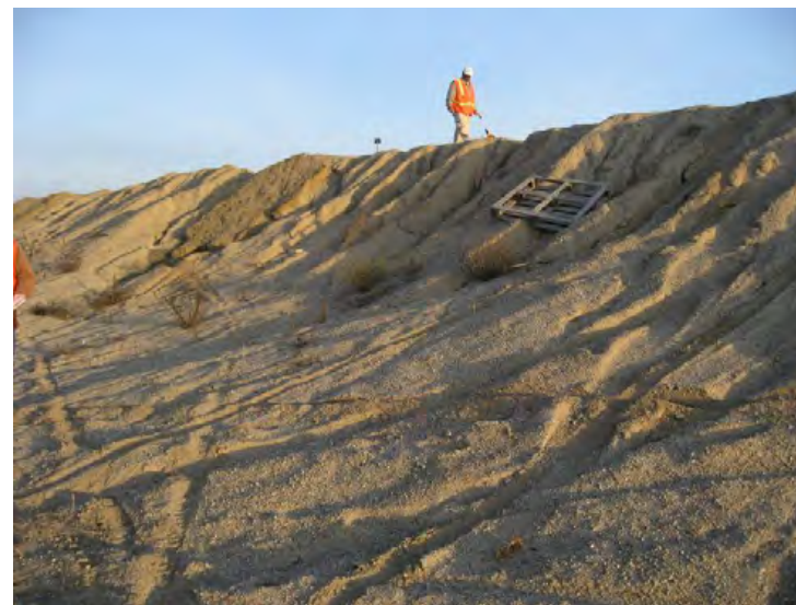
Santa Clara River Levee, From Hwy 101 to Saticoy. (Photo No. M15) – Erosion of levee embankment, looking upstream (riverward side)
