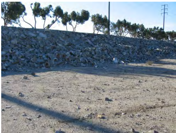
Santa Clara River Levee, From Hwy 101 to Saticoy. (Photo No. M26) – Concrete pipe debris along levee toe, looking d/s (riverward side)
