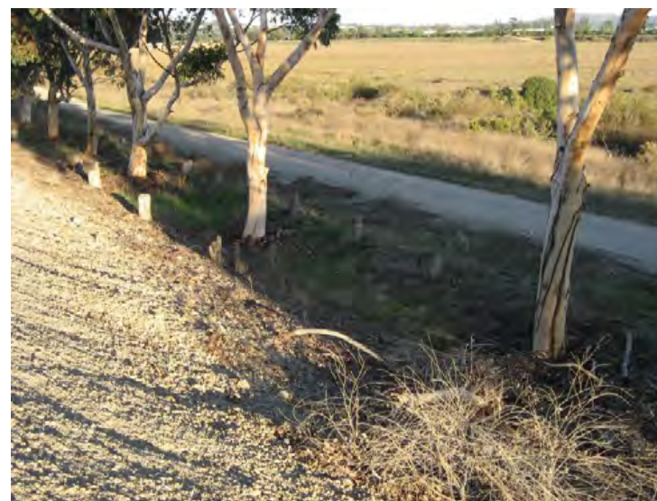
Santa Clara River Levee, From Hwy 101 to Saticoy, (Photo No. M59) – Trees within 15' of levee toe, looking u/s (landward side)
