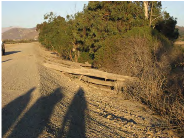
Santa Clara River Levee, From Hwy 101 to Saticoy, (Photo No. M65) – Trees and fallen trees within 15' of levee toe, looking u/s (landward side)
