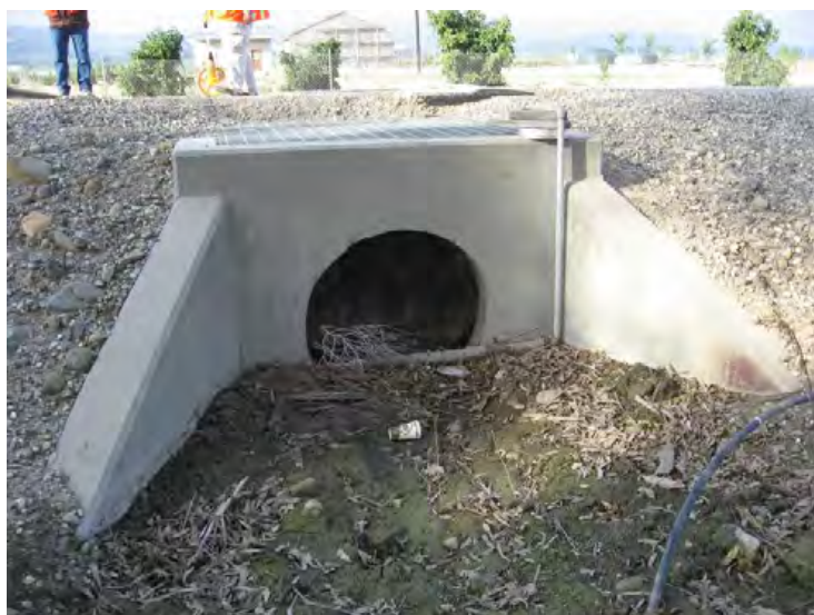
Santa Clara River Levee, From Hwy 101 to Saticoy. (Photo No. M5) – Sediment deposition in Side Drain No. 1, 42” RCP inlet (landward side)
