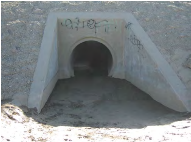
Santa Clara River Levee, From Hwy 101 to Saticoy. (Photo No. M29) – Sediment deposition in Side Drain No. 6, 48" RCP outlet (riverward side)
