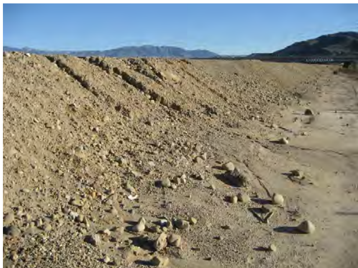
Santa Clara River Levee, From Hwy 101 to Saticoy, (Photo No. M73) – Erosion on levee embankment, looking upstream (landward side)
