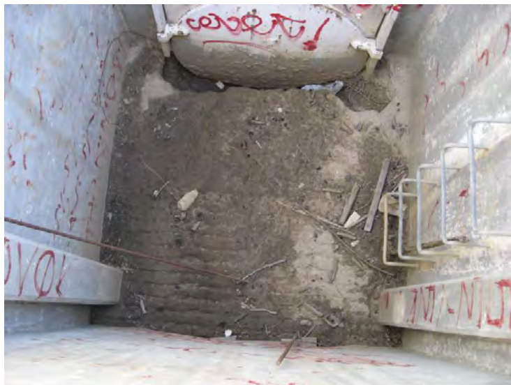
Santa Clara River Levee, From Hwy 101 to Saticoy, (Photo No. M50) – Looking down at sediment in SD No. 4, inlet structure (landward side)
