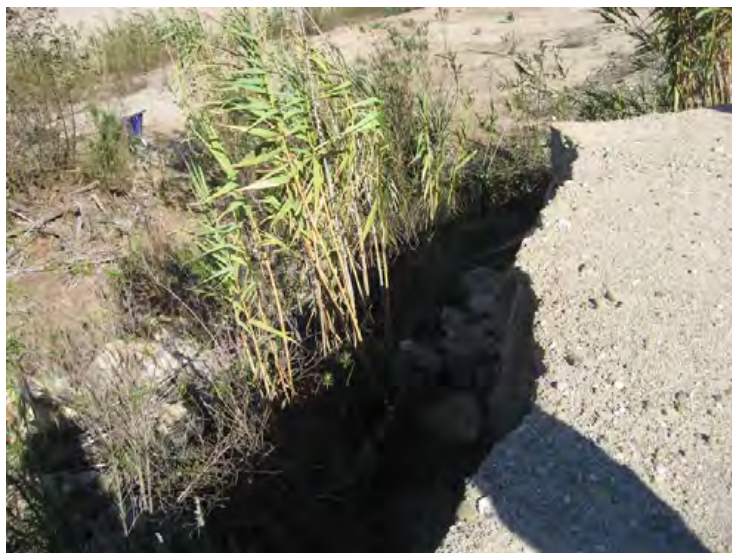
Santa Clara River Levee, From Hwy 101 to Saticoy. (Photo No. M33) – Exposure of tip of buried groin looking downstream (riverward side)
