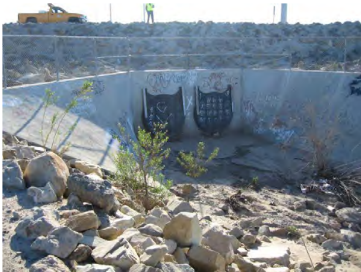
Santa Clara River Levee, From Hwy 101 to Saticoy. (Photo No. P6) – Central Avenue Drain, 2-72” RCP with flap gates (riverward side)
