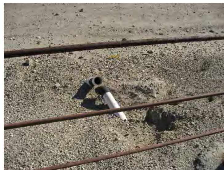
Santa Clara River Levee, From Hwy 101 to Saticoy, (Photo No. M43) – PVC pipe protruding from levee (landward side)
