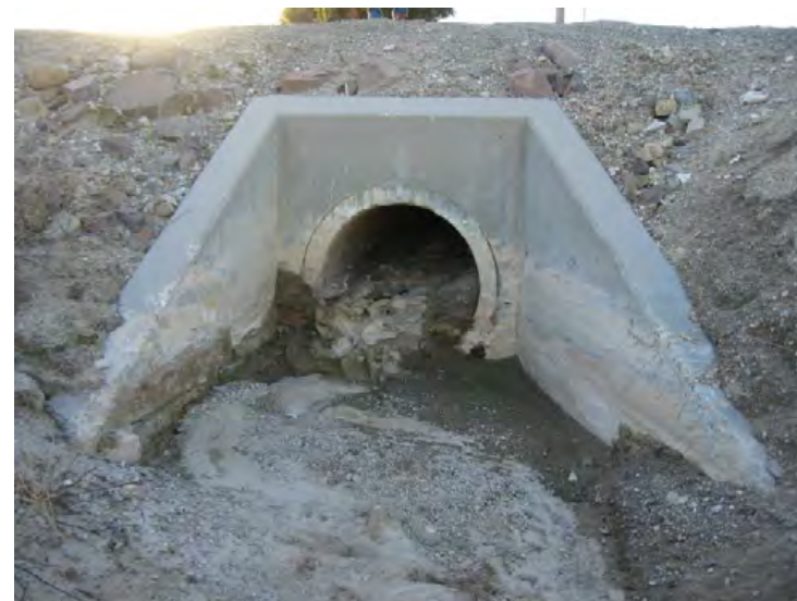
Santa Clara River Levee, From Hwy 101 to Saticoy. (Photo No. M20) – Sediment deposition in Side Drain No. 3, 48" RCP outlet (riverward side)
