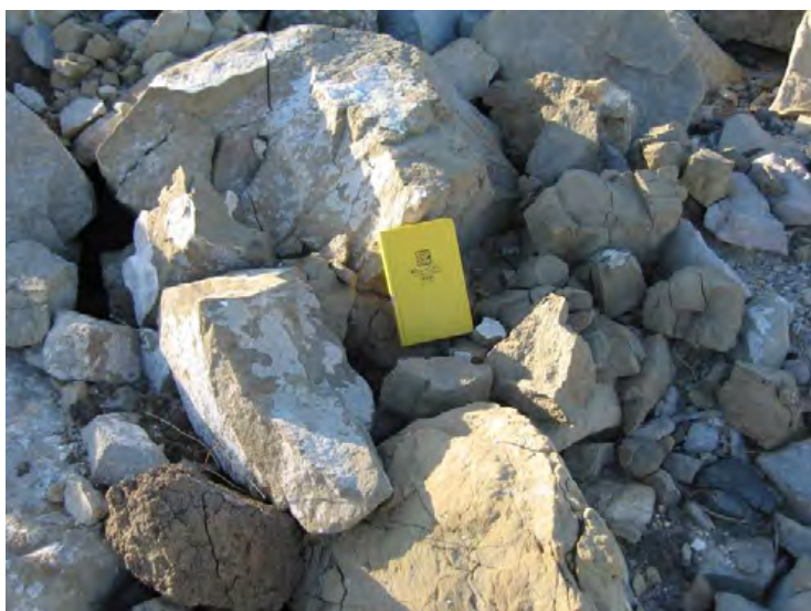
Santa Clara River Levee, From Hwy 101 to Saticoy. (Photo No. M25) – Broken stone revetment (riverward side)
