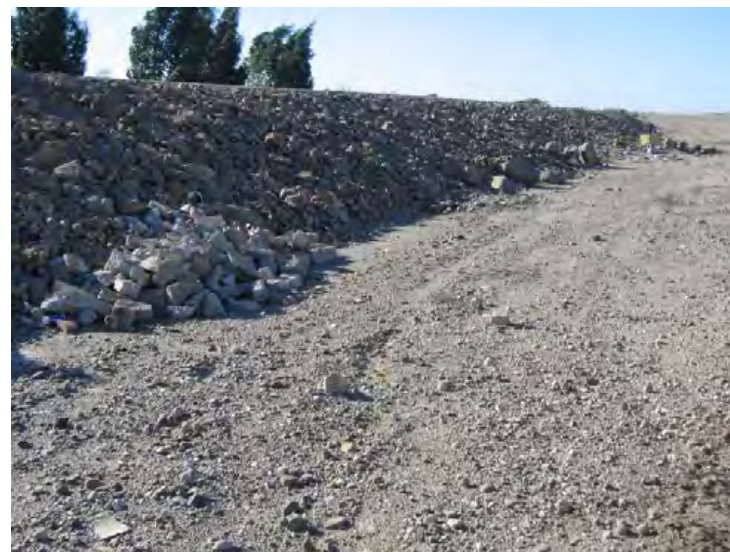
Santa Clara River Levee, From Hwy 101 to Saticoy. (Photo No. M28) – Debris along levee toe, looking downstream (riverward side)
