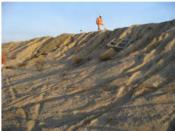
Santa Clara River Levee, From Hwy 101 to Saticoy. (Photo No. M17) – Erosion of levee embankment, adjacent to asphalt plant (riverward side)
