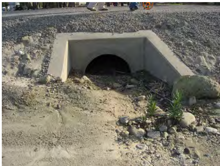
Santa Clara River Levee, From Hwy 101 to Saticoy. (Photo No. P2) – Side Drain No. 1, 42\"/>
