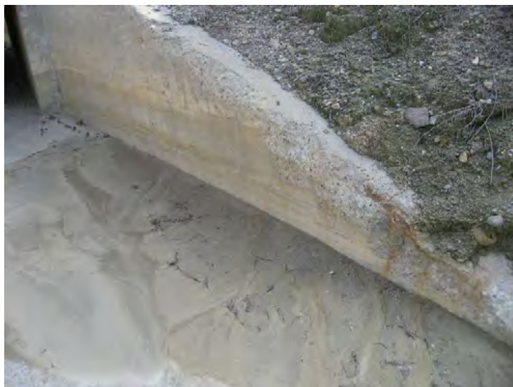
Santa Clara River Levee, From Hwy 101 to Saticoy. (Photo No. M2) – Detail of damaged concrete headwall & exposed rebar (riverward side)
