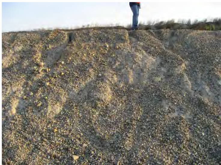
Santa Clara River Levee, From Hwy 101 to Saticoy. (Photo No. M14) – Erosion on levee embankment, looking d/s (riverward side)
