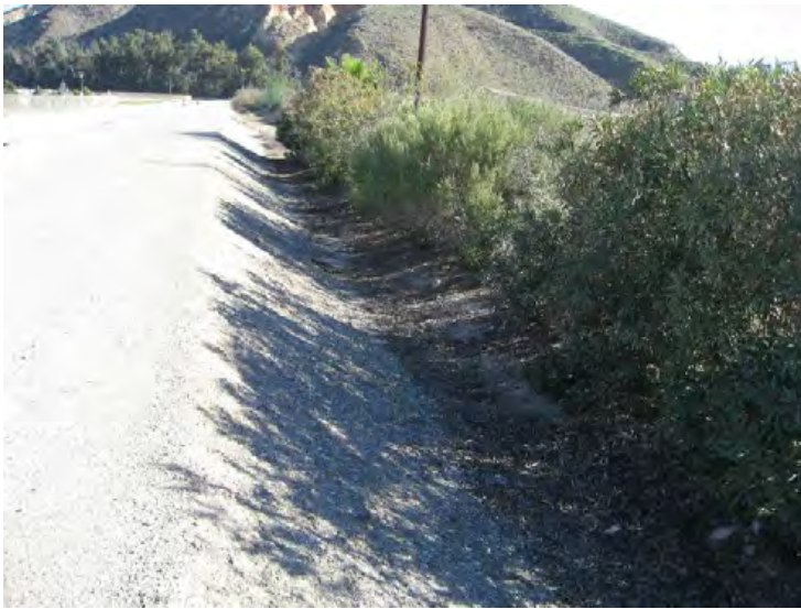
Santa Clara River Levee, From Hwy 101 to Saticoy, (Photo No. M81) – Vegetation within 15-feet of levee toe, looking upstream (landward side)
