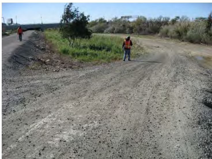
Santa Clara River Levee, From Hwy 101 to Saticoy. (Photo No. M41) – Vegetation within 15' levee toe, looking d/s (riverward side)
