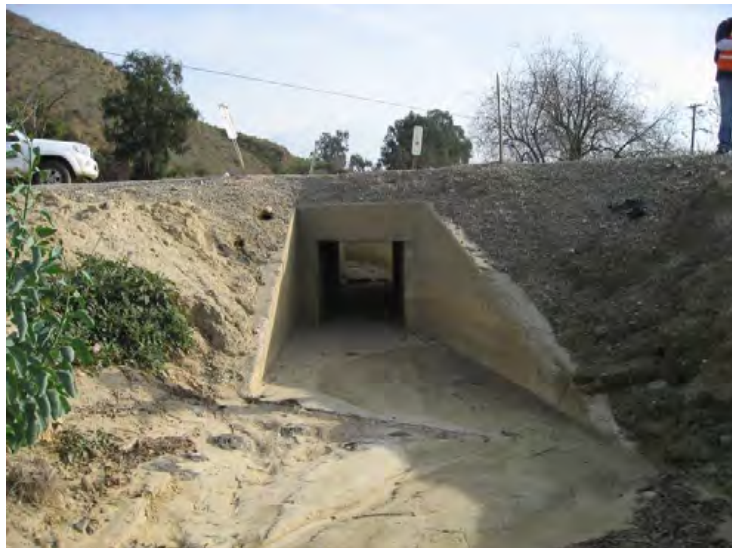
Santa Clara River Levee, From Hwy 101 to Saticoy. (Photo No. P1 – Side drain 1-A, 4' x 4' R.C.B located at upstream end of levee (riverward side)
