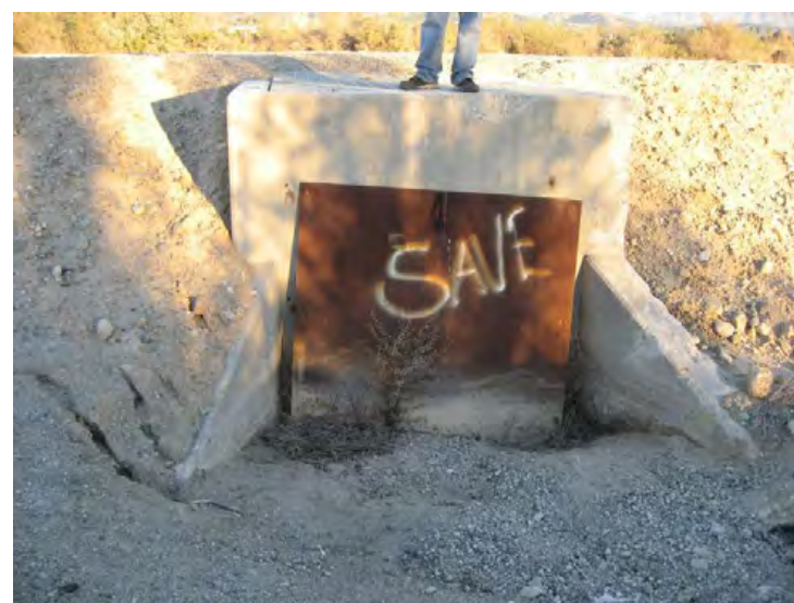
Santa Clara River Levee, From Hwy 101 to Saticoy, (Photo No. M71) – Sediment & metal debris in Side Drain No. 3 inlet (landward side)
