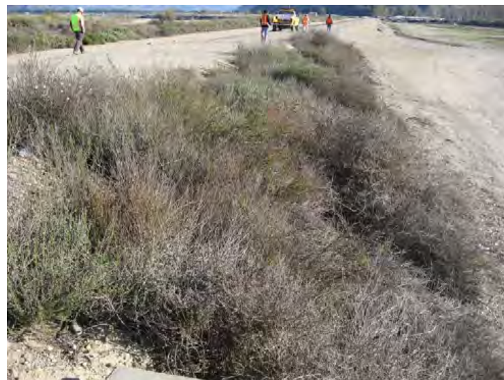
Santa Clara River Levee, From Hwy 101 to Saticoy, (Photo No. M76) – Vegetation within 15-feet of levee toe, looking downstream (landward side)
