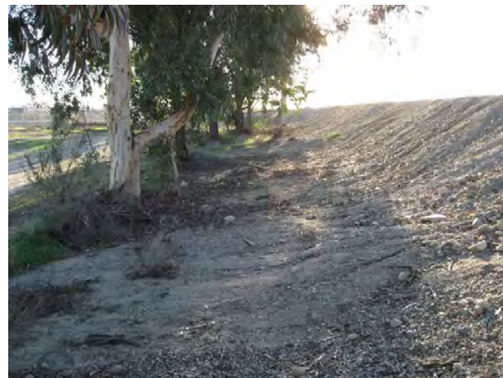
Santa Clara River Levee, From Hwy 101 to Saticoy, (Photo No. M56) – Trees within 15' of levee toe, looking upstream (landward side)
