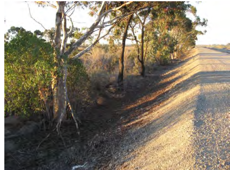
Santa Clara River Levee, From Hwy 101 to Saticoy, (Photo No. M68) – Vegetation within 15-feet of levee toe, looking d/s (landward side)
