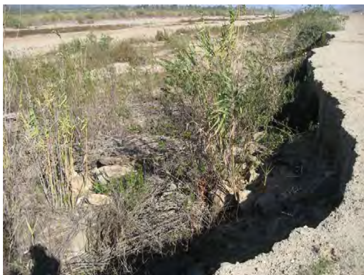
Santa Clara River Levee, From Hwy 101 to Saticoy. (Photo No. M37) – Exposure of tip of buried groin, looking upstream (riverward side)
