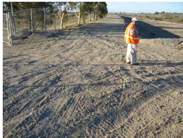
Santa Clara River Levee, From Hwy 101 to Saticoy. (Photo No. M23) – Erosion on top of levee caused by vehicles, looking d/s (riverward side)
