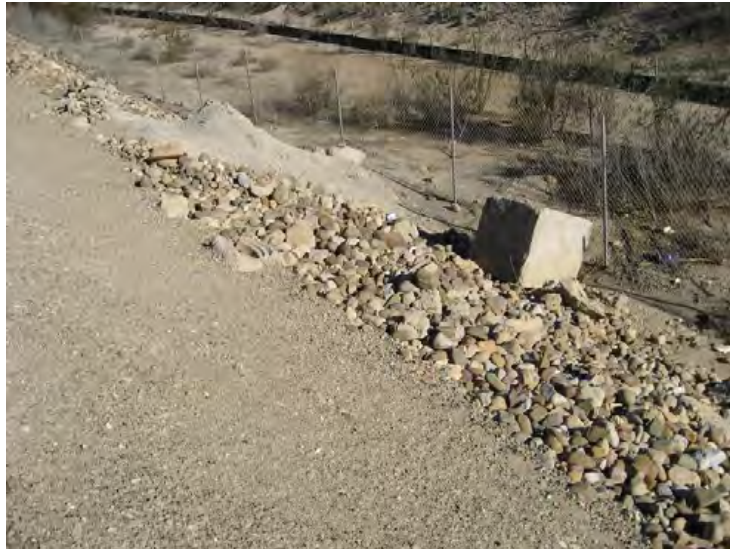
Santa Clara River Levee, From Hwy 101 to Saticoy, (Photo No. M45) – Stone debris approx. 500' along levee toe, looking u/s (landward side)
