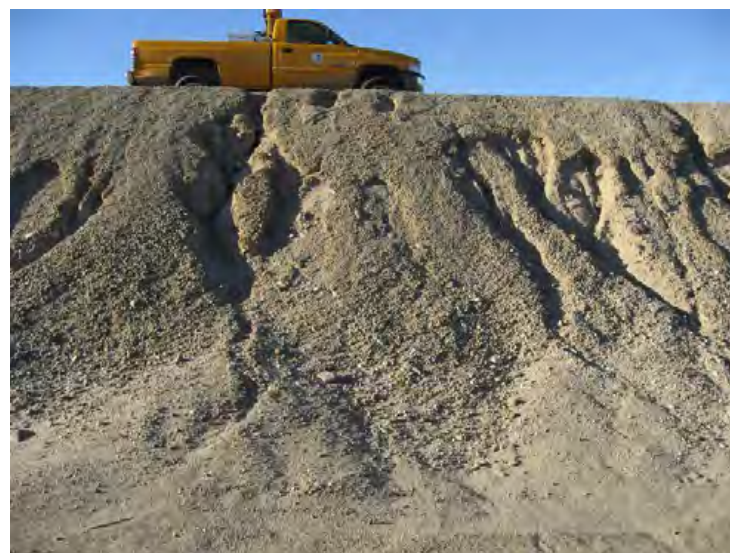
Santa Clara River Levee, From Hwy 101 to Saticoy, (Photo No. M51) – Erosion on levee embankment, looking upstream (landward side)
