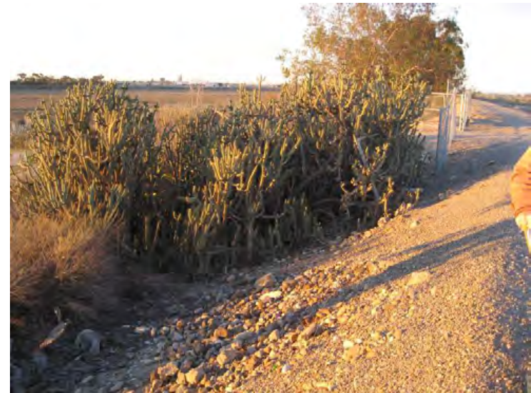
Santa Clara River Levee, From Hwy 101 to Saticoy, (Photo No. M67) – Vegetation within 15-feet of levee toe, looking downstream (landward side)
