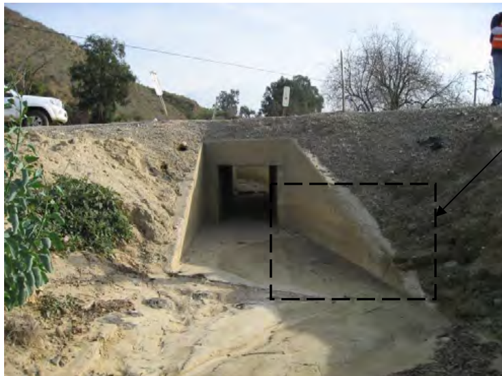
Santa Clara River Levee, From Hwy 101 to Saticoy. (Photo No. M1) – Damaged concrete on Side Drain 1A headwall with rebar exposed
