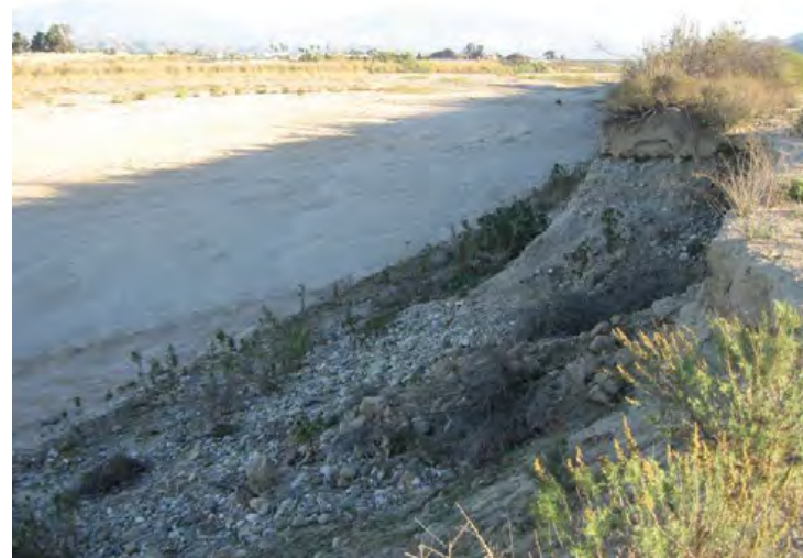
Santa Clara River Levee, From Hwy 101 to Saticoy. (Photo No. F2) – 20' -25' high erosion cut eroding towards levee, looking u/s (riverward)
