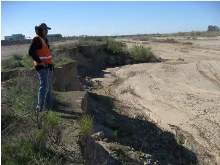
Santa Clara River Levee, From Hwy 101 to Saticoy. (Photo No. F3) – Erosion cut eroding towards levee exposing groins, looking d/s (riverward)
