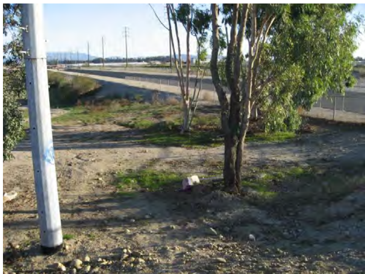
Santa Clara River Levee, From Hwy 101 to Saticoy, (Photo No. M54) – Tree within 15' of levee toe, looking downstream (landward side)
