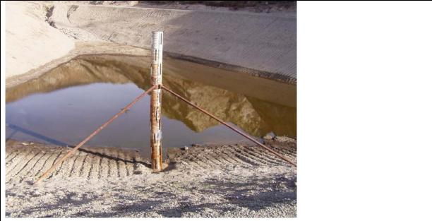
Real Wash Debris Basin- Zone 2. Perforated CMP Debris Bleeder Riser Tower
