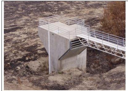
Las Lllajas Detention Basin- Zone 3. Operating Spillway, Reinforced Concrete Two-Way Riser Tower with Projecting Top and Side Inlets with Trash Rack
