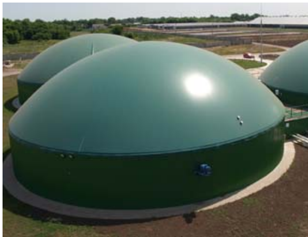
Figure 5-6 Example – Storage Tanks with Membrane Biogas Holding Roof
