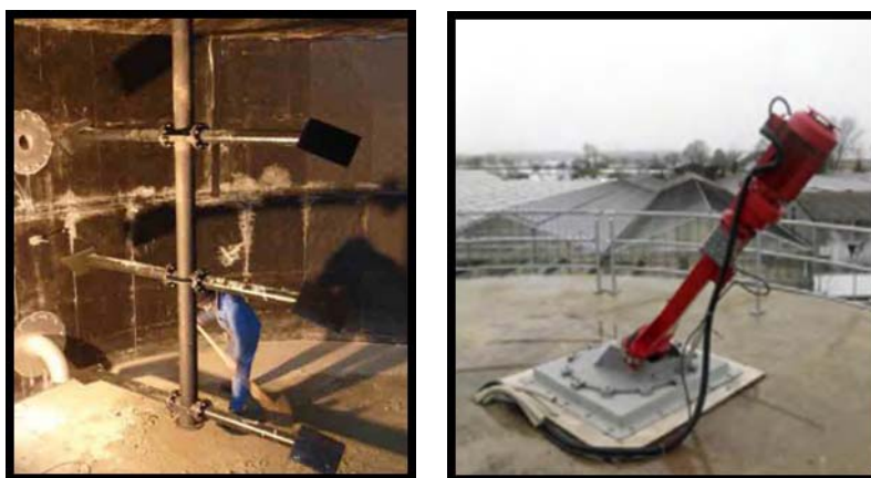
Figure 4-6 Kolbermoor AD Paddle Mixer
