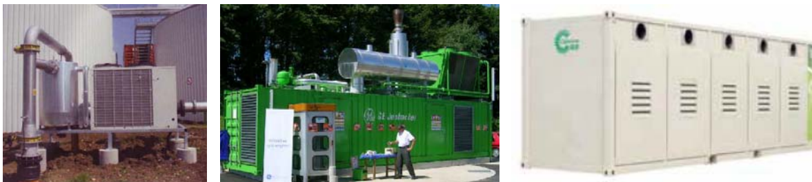
Figure 5-8 Examples - Condensate Trap/Cooling Unit (left); ICE CHP (middle); Microturbine CHP Package (right)
