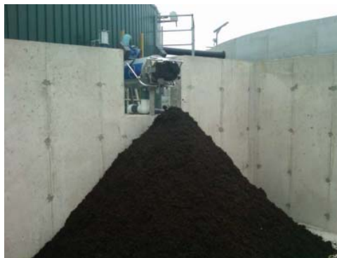
Figure 5-7 Example – Solid-Liquid-Separation with Discharged Solids
