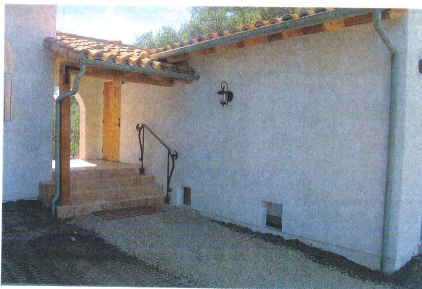
FRONT VIEW BREEZEWAY, TOWER & STEPS NOTE FLOOD VENT OPENINGS INTO GARAGE
