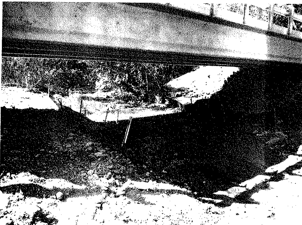
Looking from upstream side of bridge showing girder soffits. 10-4-13
