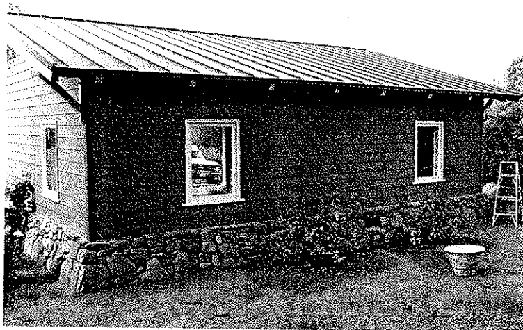
REAR - NORTH SIDE OF GARAGE
