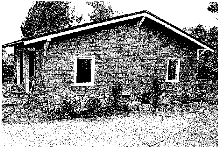
RIGHT - EAST SIDE OF GARAGE
