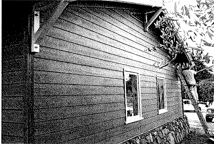
LEFT - WEST SIDE OF GARAGE
