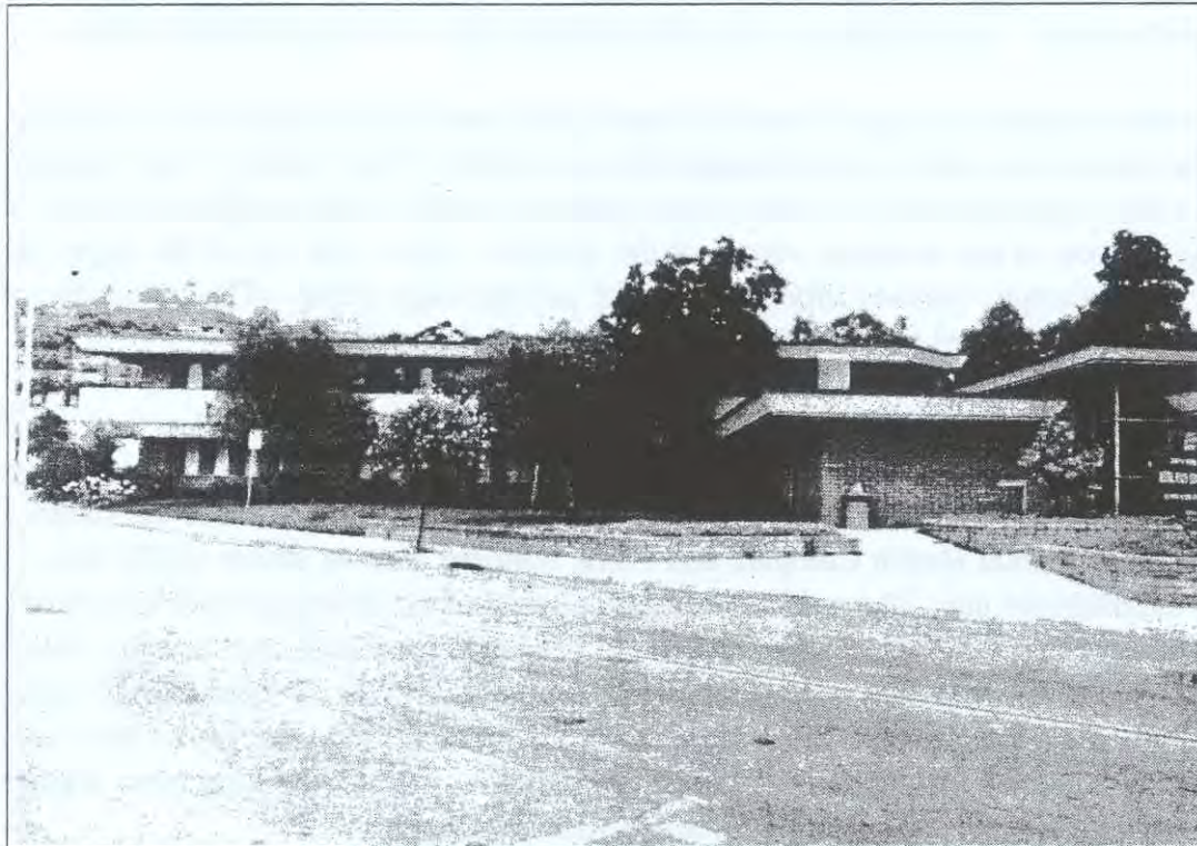
B. View of existing mental health complex from Hillmont Avenue looking northeast.
