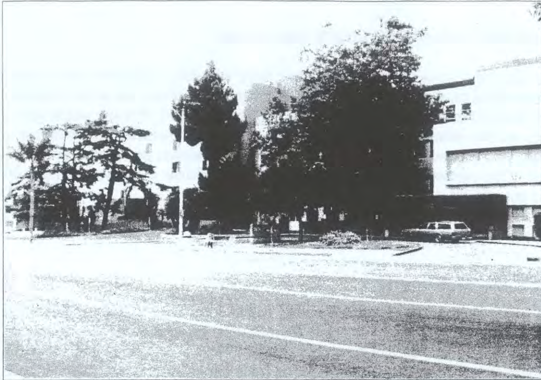
A. View of existing hospital from Loma Vista Road looking north.
