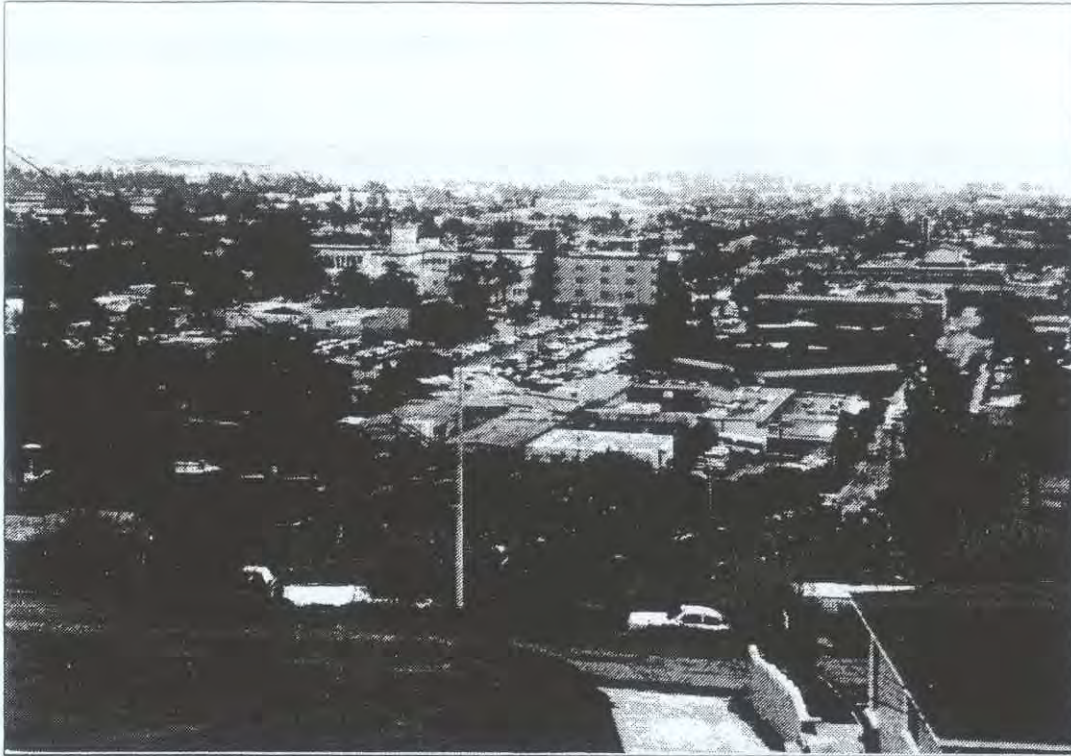
C. Existing view of the VCMC campus and uses south of the campus from 628 Whitecap Drive. Proposed project structures would be visible from this vantage point.
